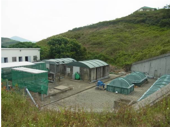
Plate 6 Existing sewage treatment plant to be upgraded
