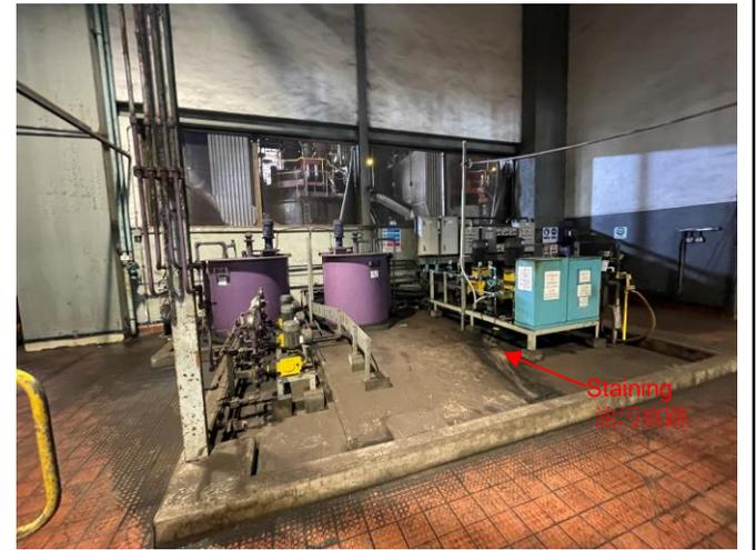
Photo 12: Chemical dosing system of unit A4 at turbine house
