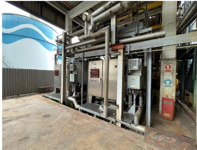
Photo 89: Sulphur melting tanks next to the sulphur store
