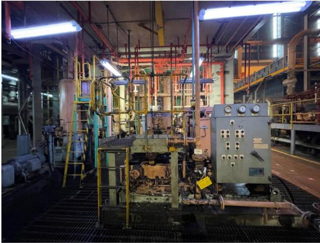
Photo 13: Seal oil system and lubrication oil system at unit A1
