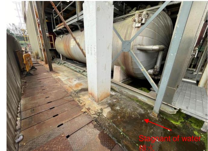
Photo 90: Sulphur melting tanks next to the sulphur store
