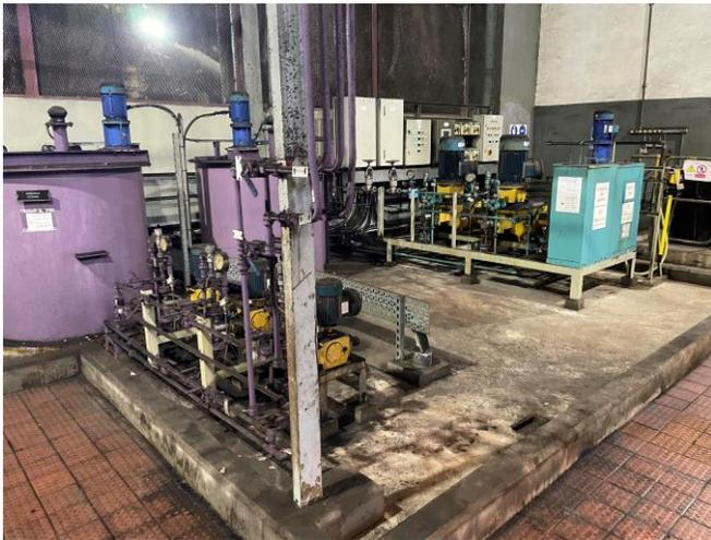
Photo 10: Chemical dosing system of unit A2 at turbine house
