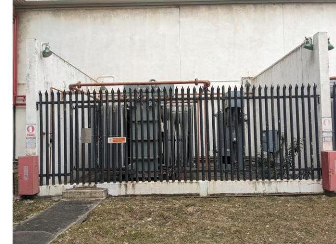
Photo 30: Unit auxiliary transformer of unit A2
