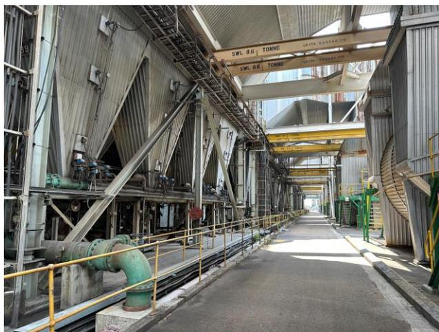
Photo 52: Electrostatic precipitator systems and induced draft fans
