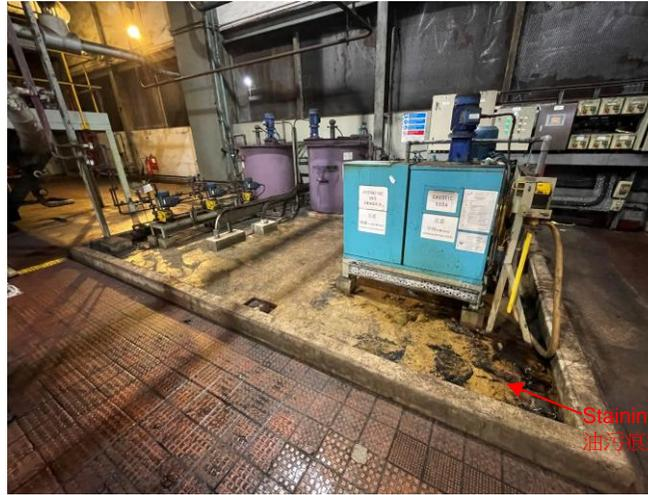
Photo 11: Chemical dosing system of unit A3 at turbine house
