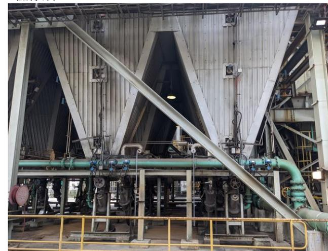
Photo 54: Electrostatic precipitator systems including ash hoppers for fly ash
