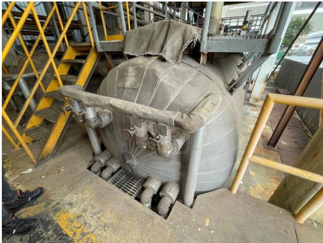
Photo 88: Sulphur melting tanks next to the sulphur store
