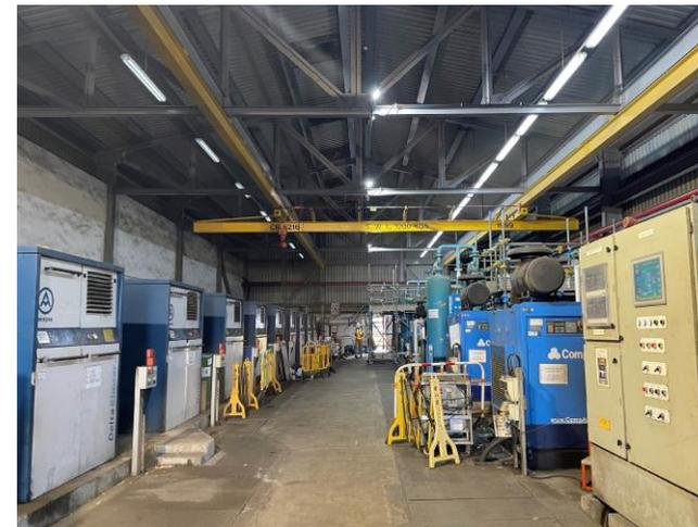
Photo 75: A compressor plant house with a series of compressors and blowers
