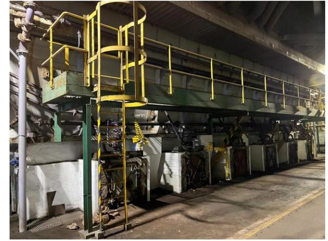
Photo 3: Ash hopper for furnace bottom ash at unit A3 inside boiler house
