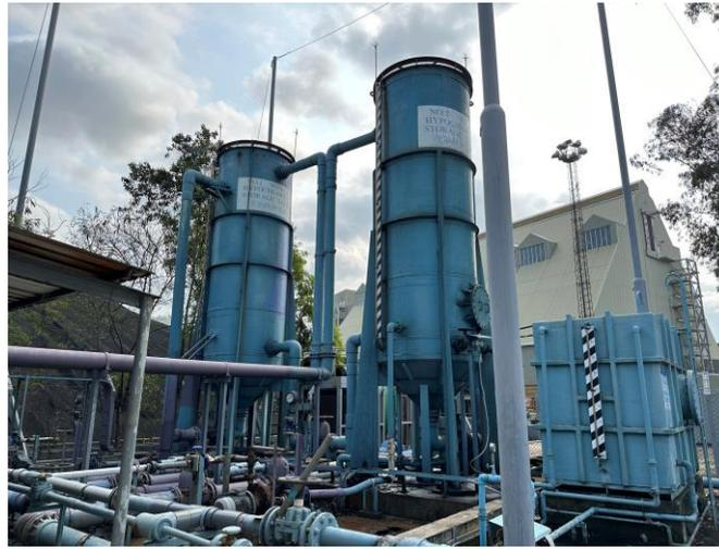
Photo 92: Two (2) aboveground tanks for storing sodium hypochlorite solution
