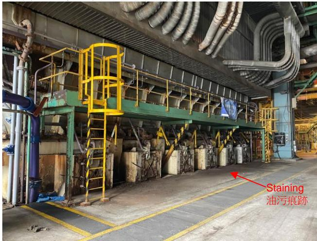
Photo 4: Ash hopper for furnace bottom ash at unit A4 inside boiler house
