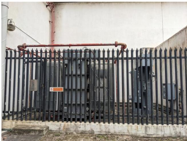
Photo 34: Unit auxiliary transformer of unit A4
