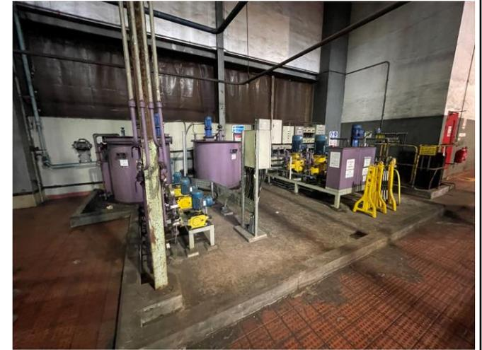
Photo 9: Chemical dosing system of unit A1 at turbine house
