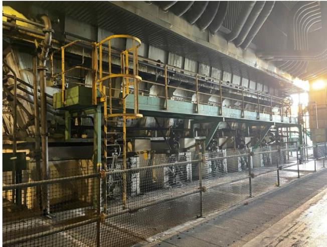
Photo 1: Ash hopper for furnace bottom ash at unit A1 inside boiler house
