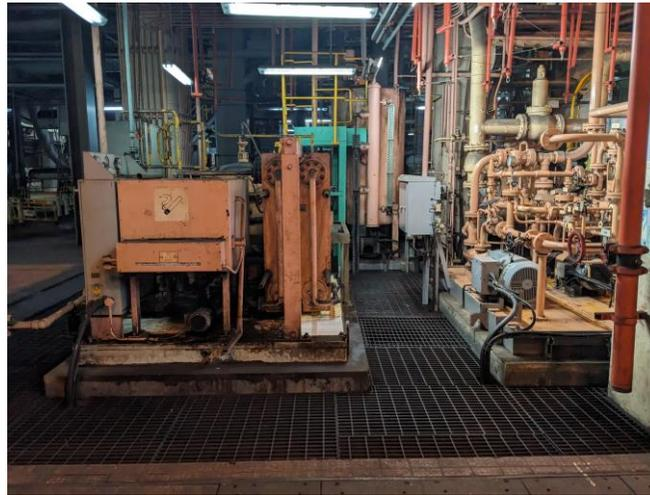
Photo 14: Seal oil system and lubrication oil system located at the drain sump
