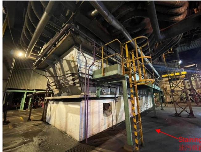
Photo 2: Ash hopper for furnace bottom ash at unit A2 inside boiler house
