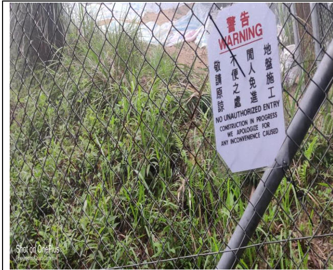
Removal of the materials on the slop
