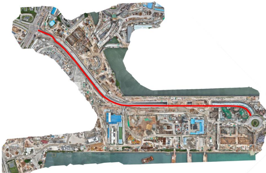
Figure 5 – New Opened Road on 31 December 2022
