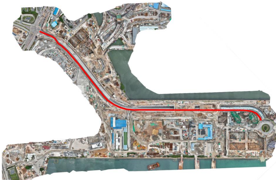
Figure 5 – New Opened Road on 31 December 2022
