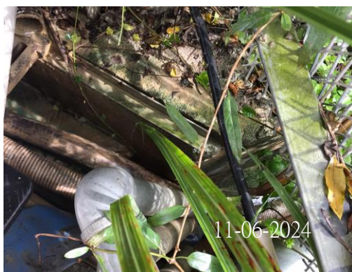
Photo 3 (Discharge point at 6/WSD)
