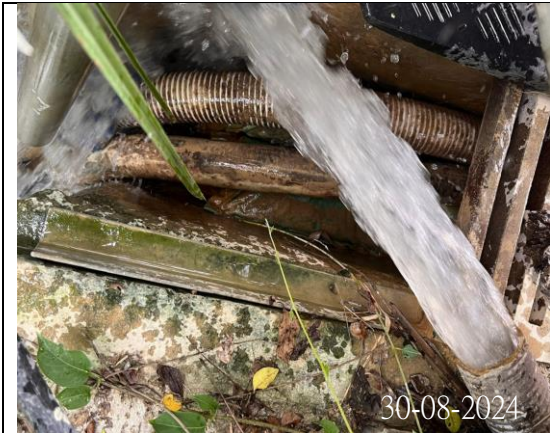
Photo 3 (Discharge point at 6/WSD)
