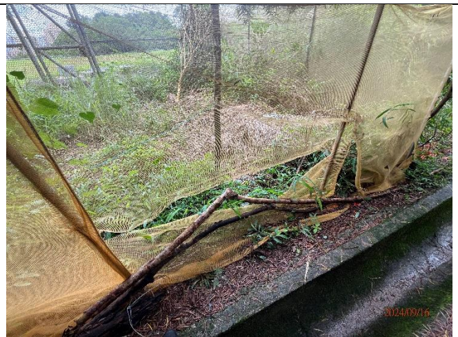
Photo 2. Protective fence of another patch of Cibotium barometz was slightly broken
