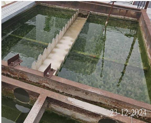
Photo 4 (Water quality of water treatment tank at 1/WSD)
