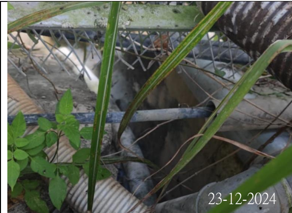
Photo 3 (Discharge point at 6/WSD)
