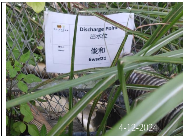
Photo 3 (Discharge point at 6/WSD)
