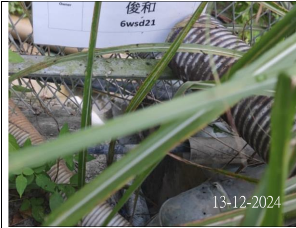
Photo 3 (Discharge point at 6/WSD)
