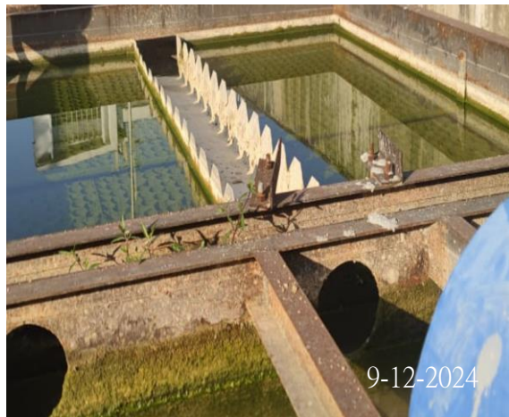
Photo 2 (Water quality of water treatment tank at 6/WSD)
