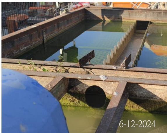
Photo 2 (Water quality of water treatment tank at 6/WSD)
