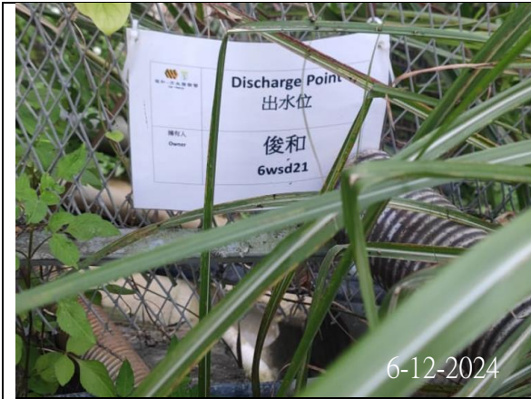
Photo 3 (Discharge point at 6/WSD)
