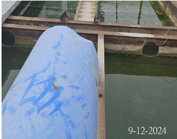
Photo 4 (Water quality of water treatment tank at 1/WSD)
