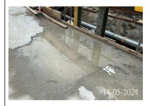
Photo 5 (Water accumulation on the site area at 1/WSD)
