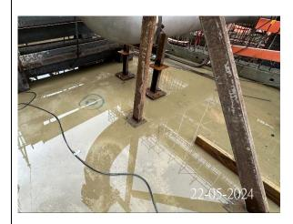
Photo 5 (Water accumulation on the site area at 1/WSD)
