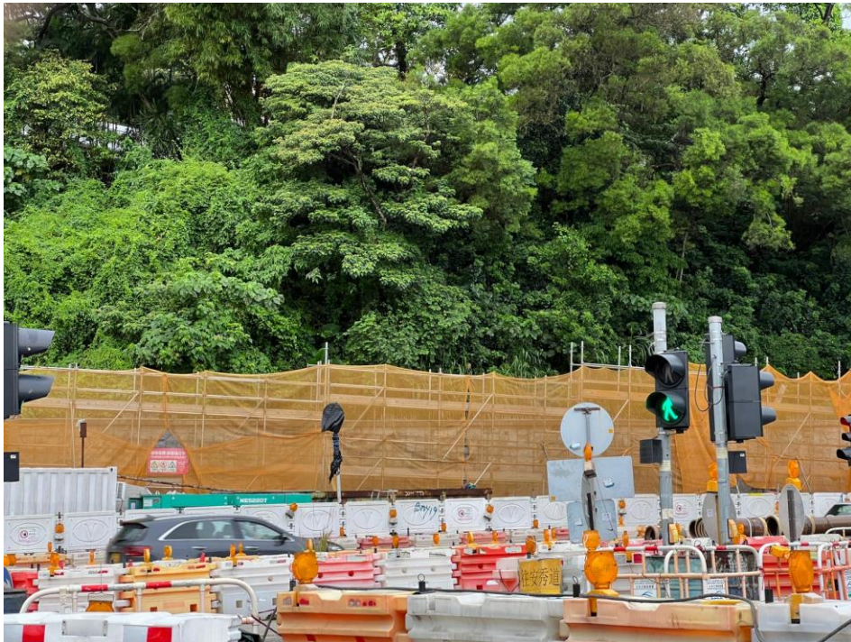
Dust netting was provided to enclose the scaffolding
