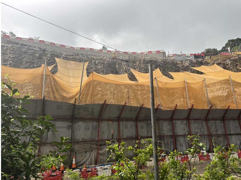
Dust netting was provided to enclose the area of dusty activities.
