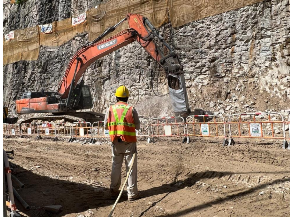
Water spraying was provided for breaking.
