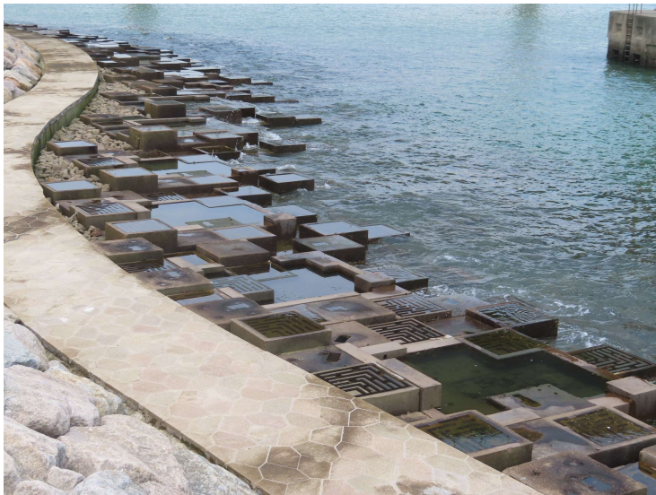
General View of Rocky Eco-shoreline
