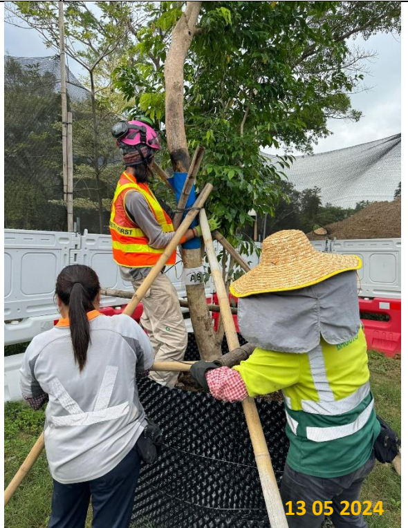
Restaking of A8 and A12 were carried out on 13 May 2024. Position of trunk protection pad was adjusted.
