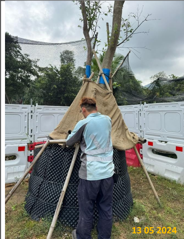
Restaking of A8 and A12 were carried out on 13 May 2024.
