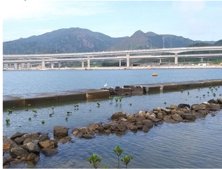
General View of Mangrove Eco-shoreline at Lower Terrace
