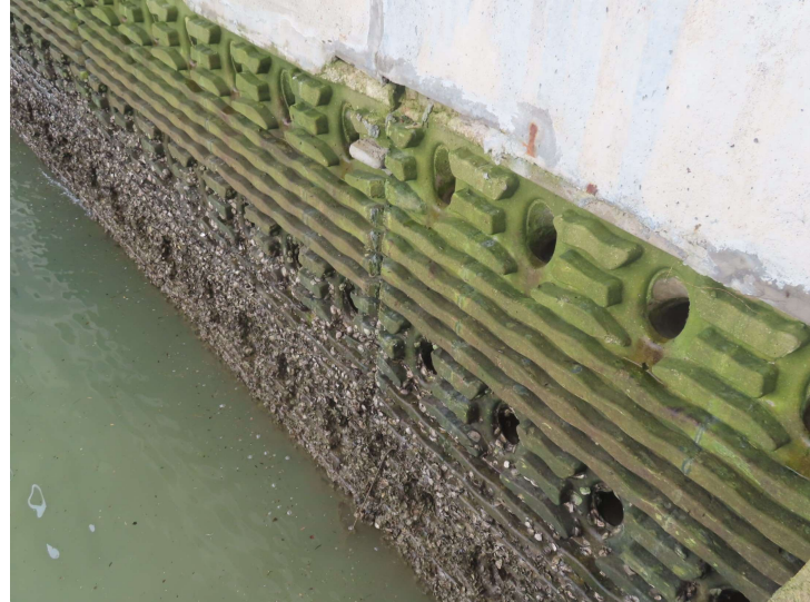
General View of Vertical Eco-shoreline
