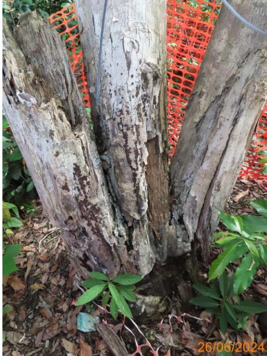
9: U041_Crack on trunk base
