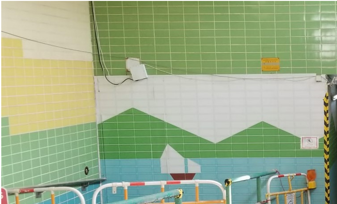
Photo 3 - Erection of site hoardings in unobtrusive colours
