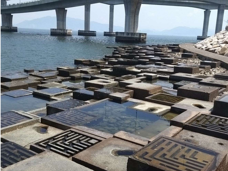
General View of Rocky Eco-shoreline
