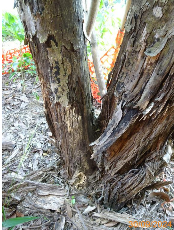
14: U041_Wood damage at trunk union#3
