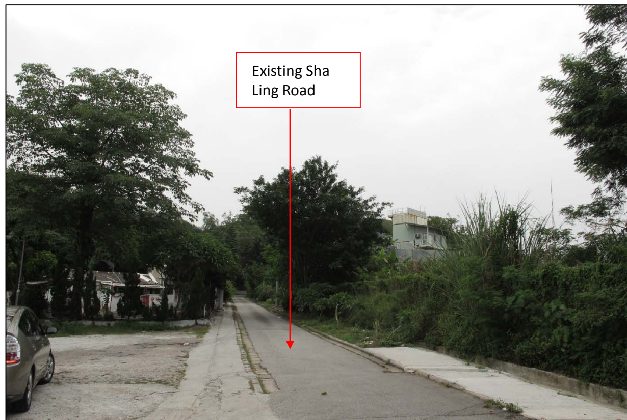
FROM VP1 EXISTING CONDITION
