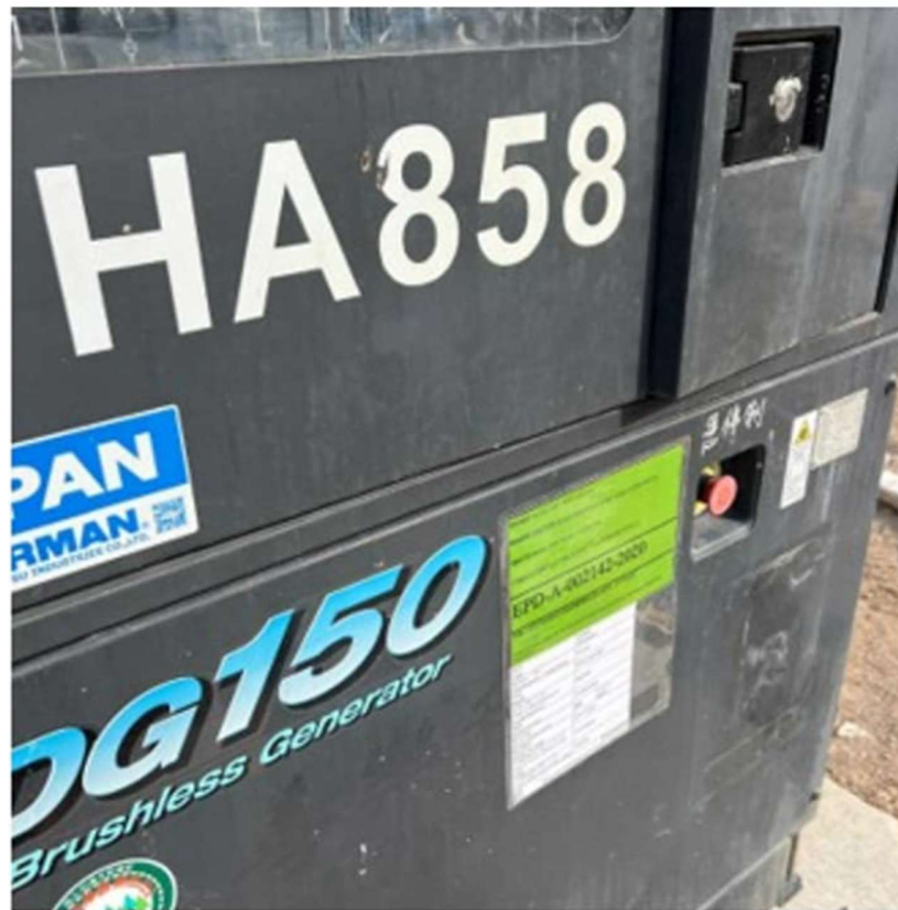
Photo 2: Power Mechanical Equipment with Quality Power Mechanical Equipment (QPME) labels were used at site to lower the noise nuisance to the nearby residents.
