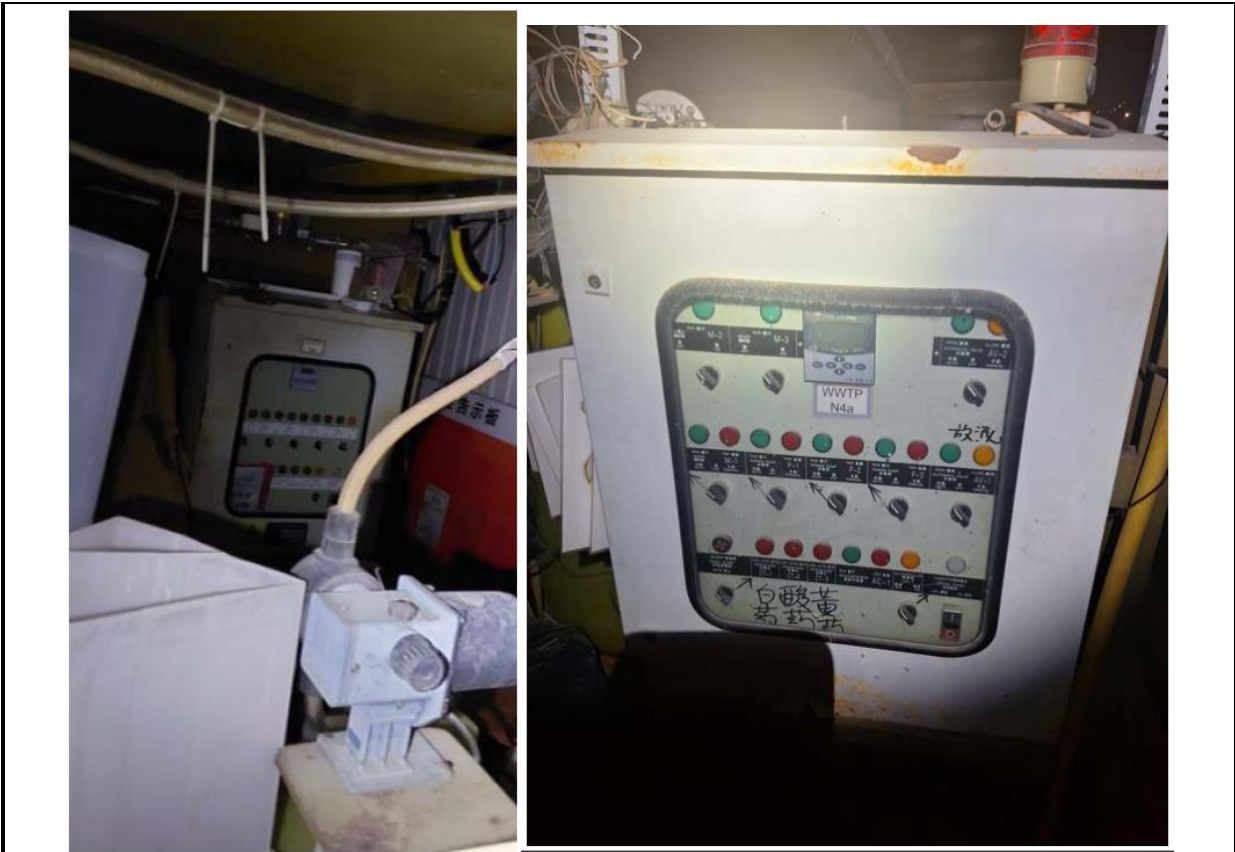
Photo 4a and 4b: Technician night shift team conduct patrol at the site area every day to ensure all unnecessary construction equipment are off.
