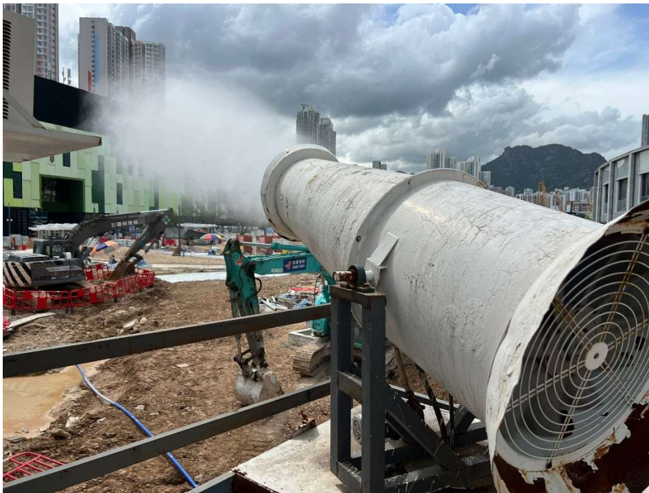
Photo 4: Water misting cannon has been provided for dust suppression on site.
