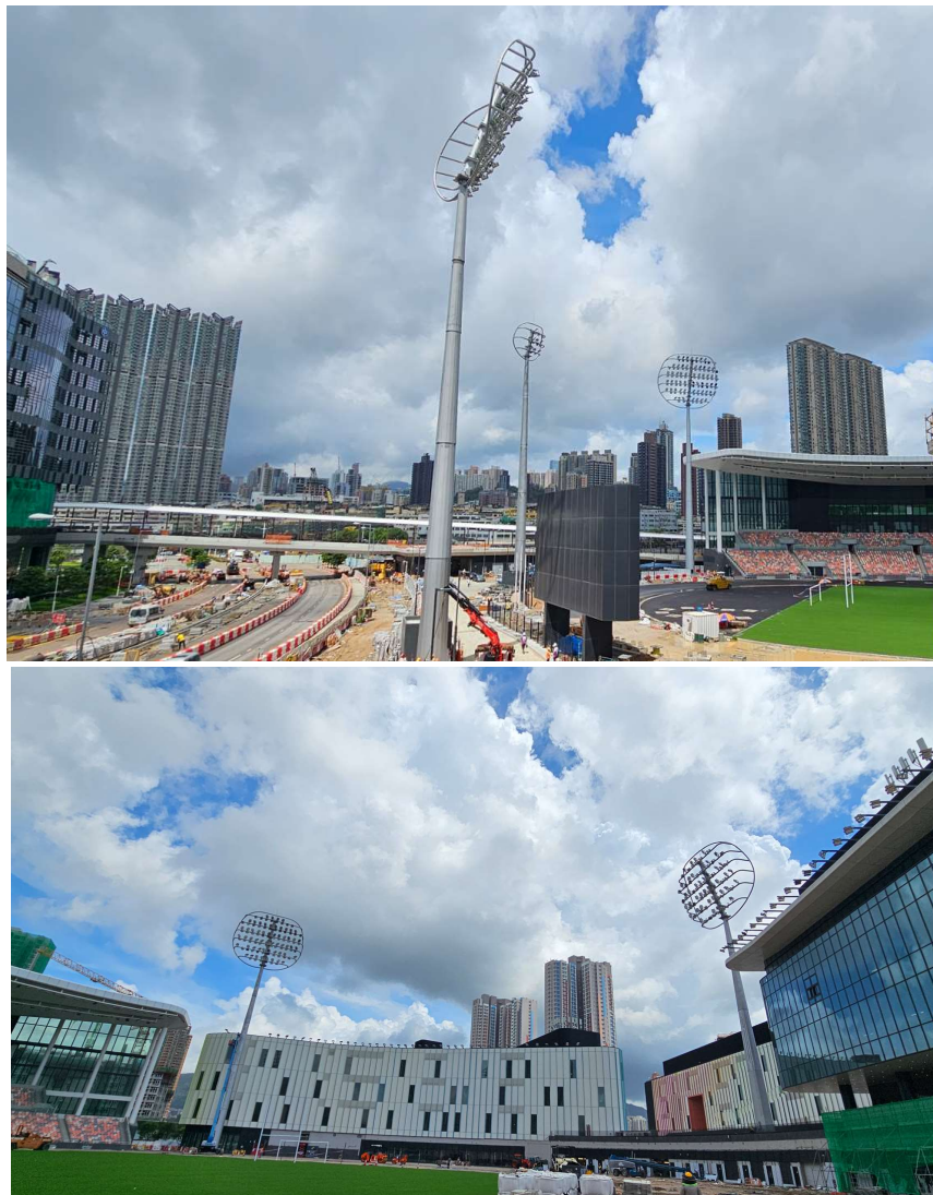
Photo 3a and 3b: Spot lights are adjusted to control lighting direction away from nearby residential.
