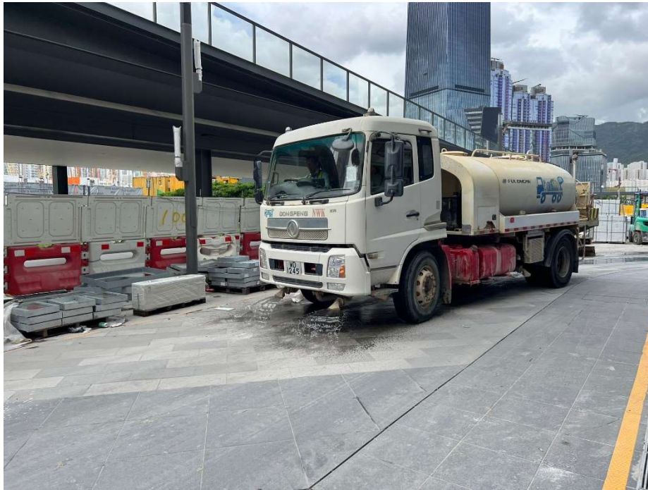
Photo 2: Water spraying truck has been provided on haul road to maintain wet surface.
