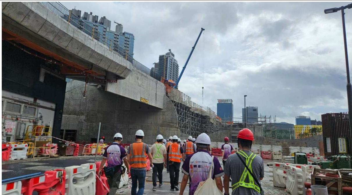
Photo 3: Regular site inspection was carried out to audit the implementation of mitigation measures on site.
