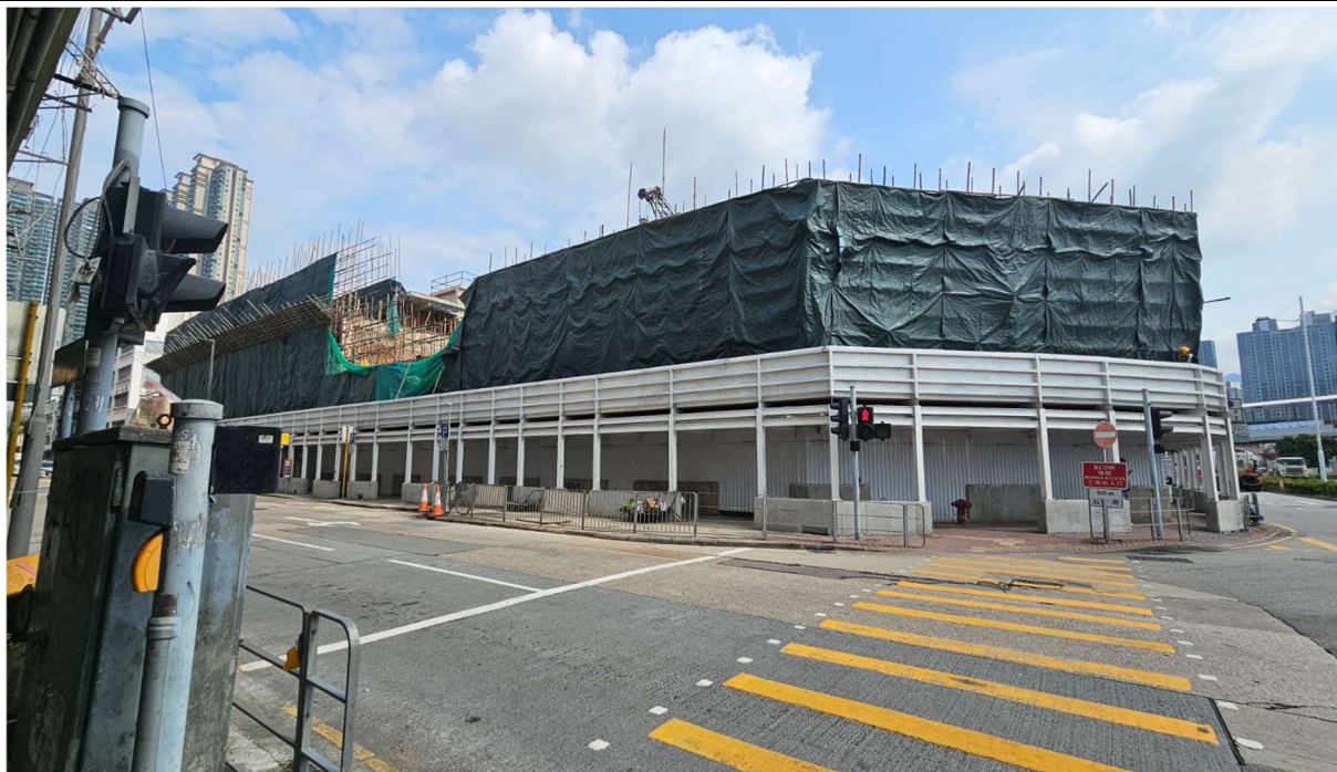
Photo 1a and 1b: Nearby demolition work at The Hong Kong Society for the Blind Workshop and Hostel on 29 August 2024.
