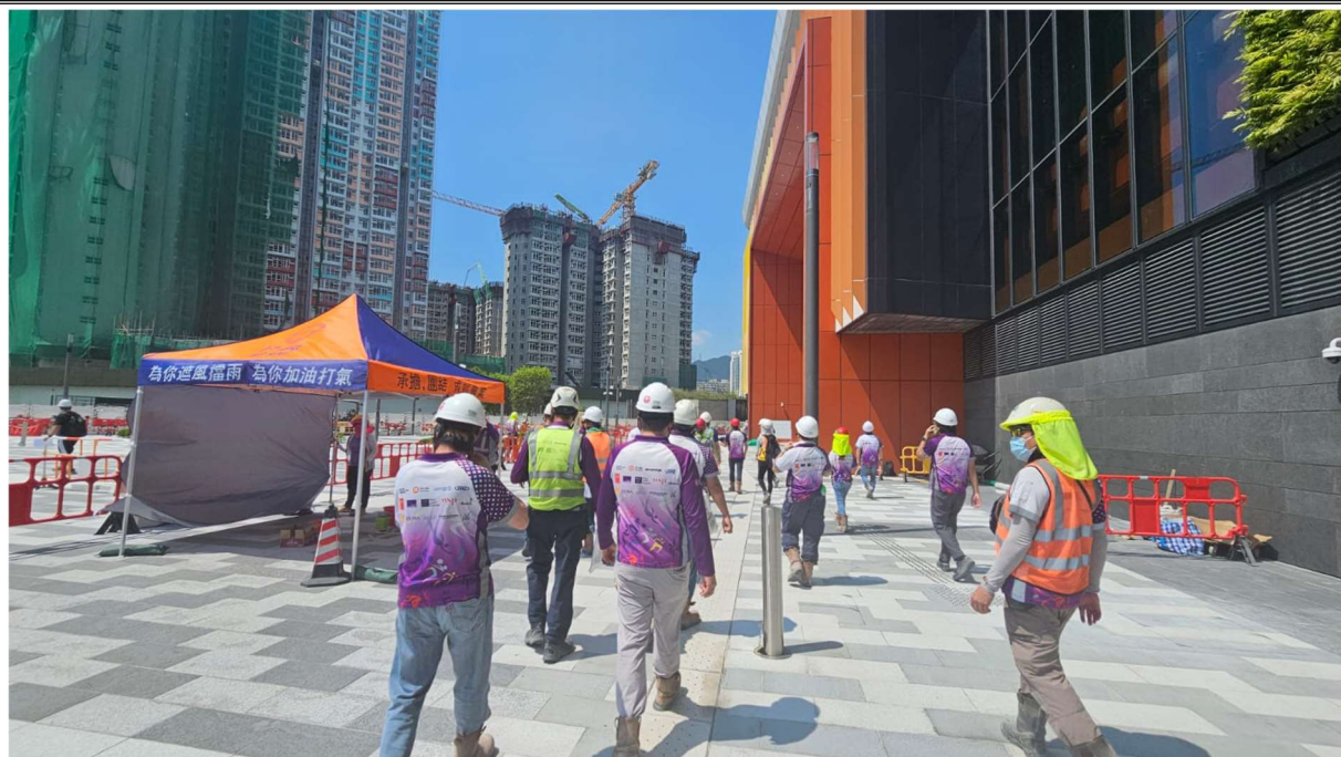
Photo 3: Regular site inspection was carried out to audit the implementation of mitigation measures on site.
