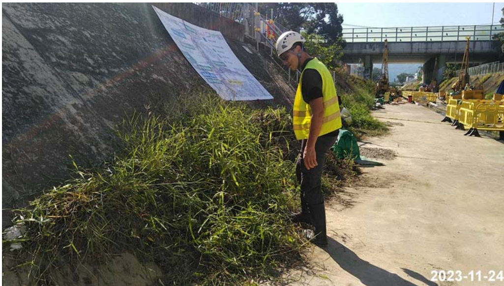
5. Direct Observation and active searching at the bottom of the embankment
