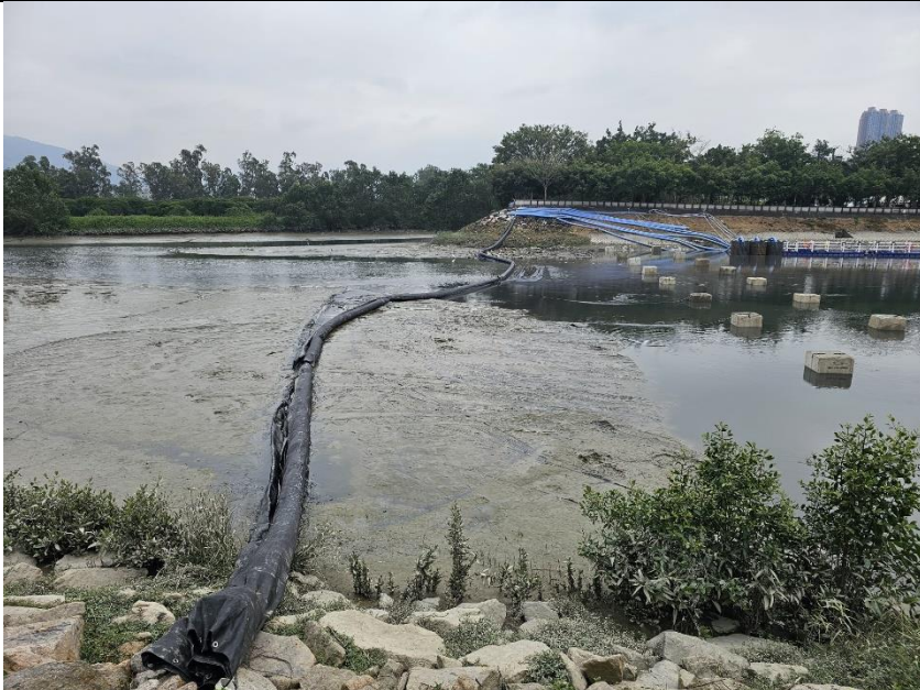
Photo 11: Preparation works for installing the inflatable dam
