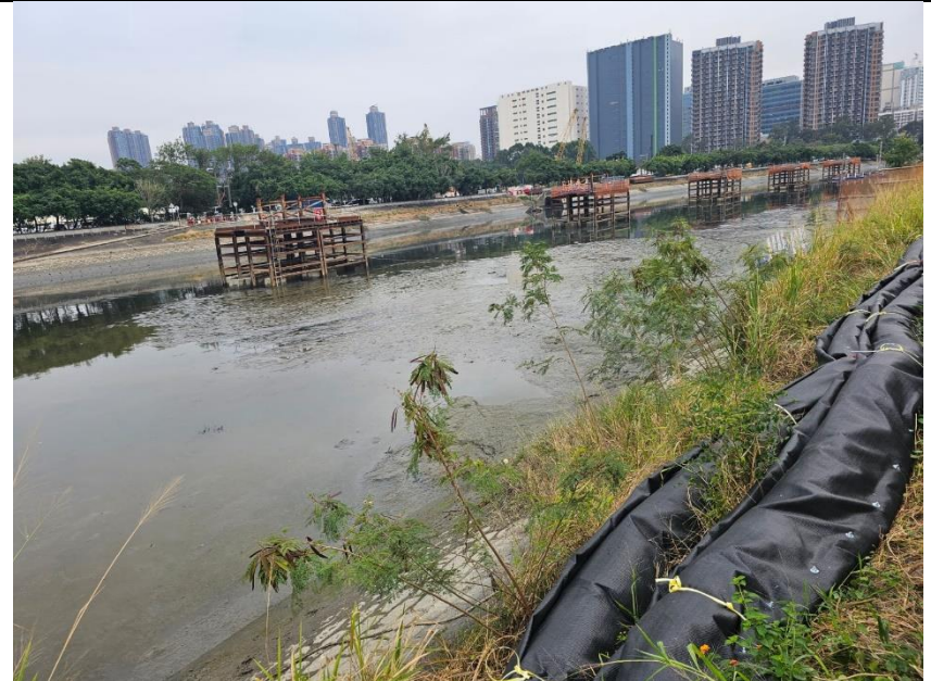
Photo 12: Platforms for conducting Ground Investigation work
