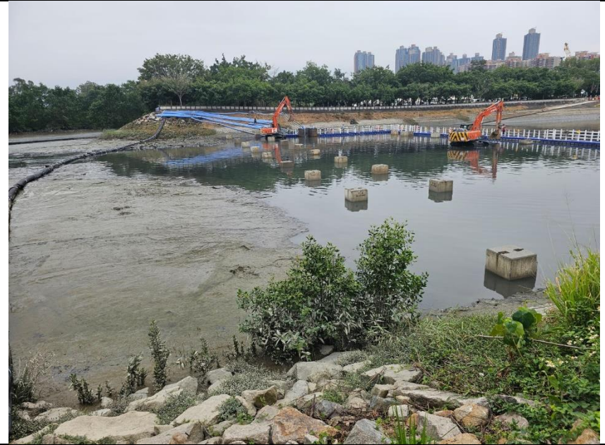
Photo 10: Preparation works for installing the inflatable dam
