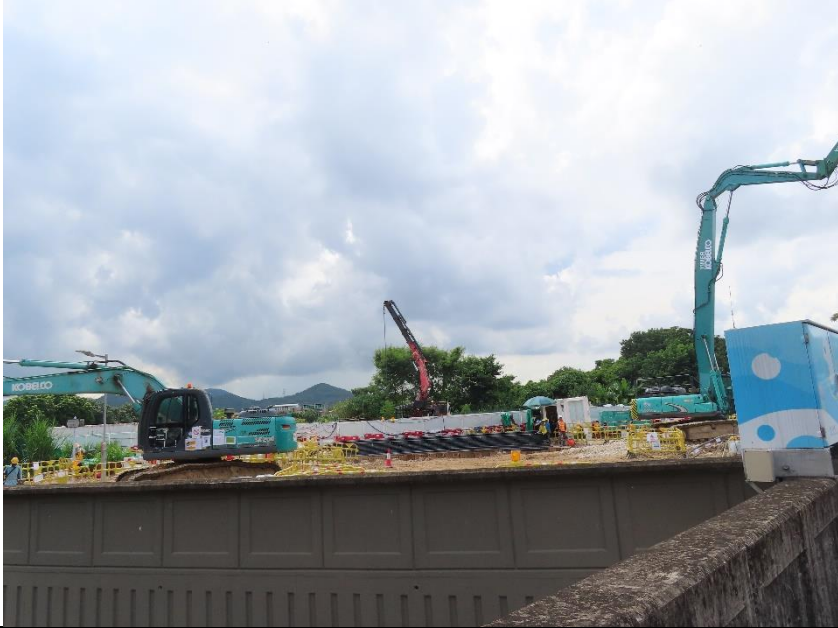
Photo 13: Construction site inside Yuen Long Town Nullah - Section 1
