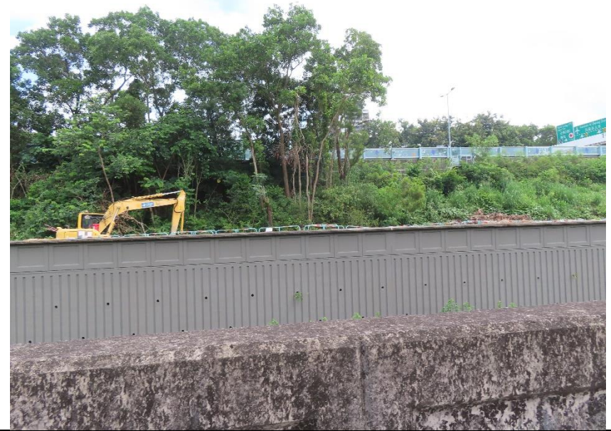
Photo 14: Construction site inside Yuen Long Town Nullah - Section 1
