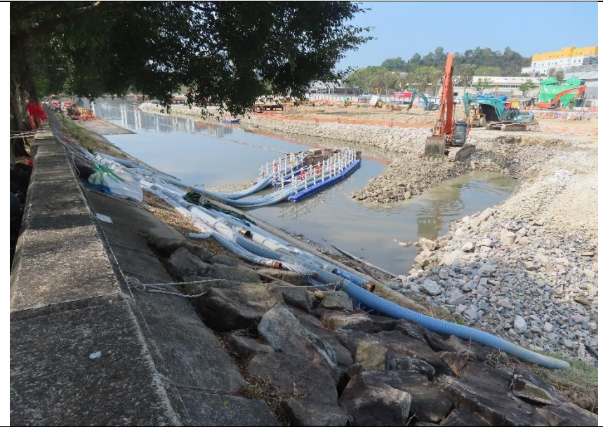
Photo 10: Platforms in Yuen Long Town Nullah - Section 4
