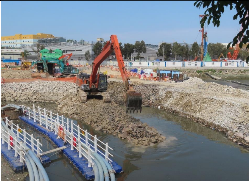
Photo 9: Preparation works for installing the inflatable dam
