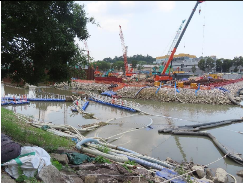
Photo 9: Sheet piling cofferdam construction at section 4 of the Yuen Long Town Nullah
