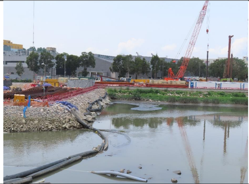
Photo 10: Sheet piling cofferdam construction at section 4 of the Yuen Long Town Nullah
