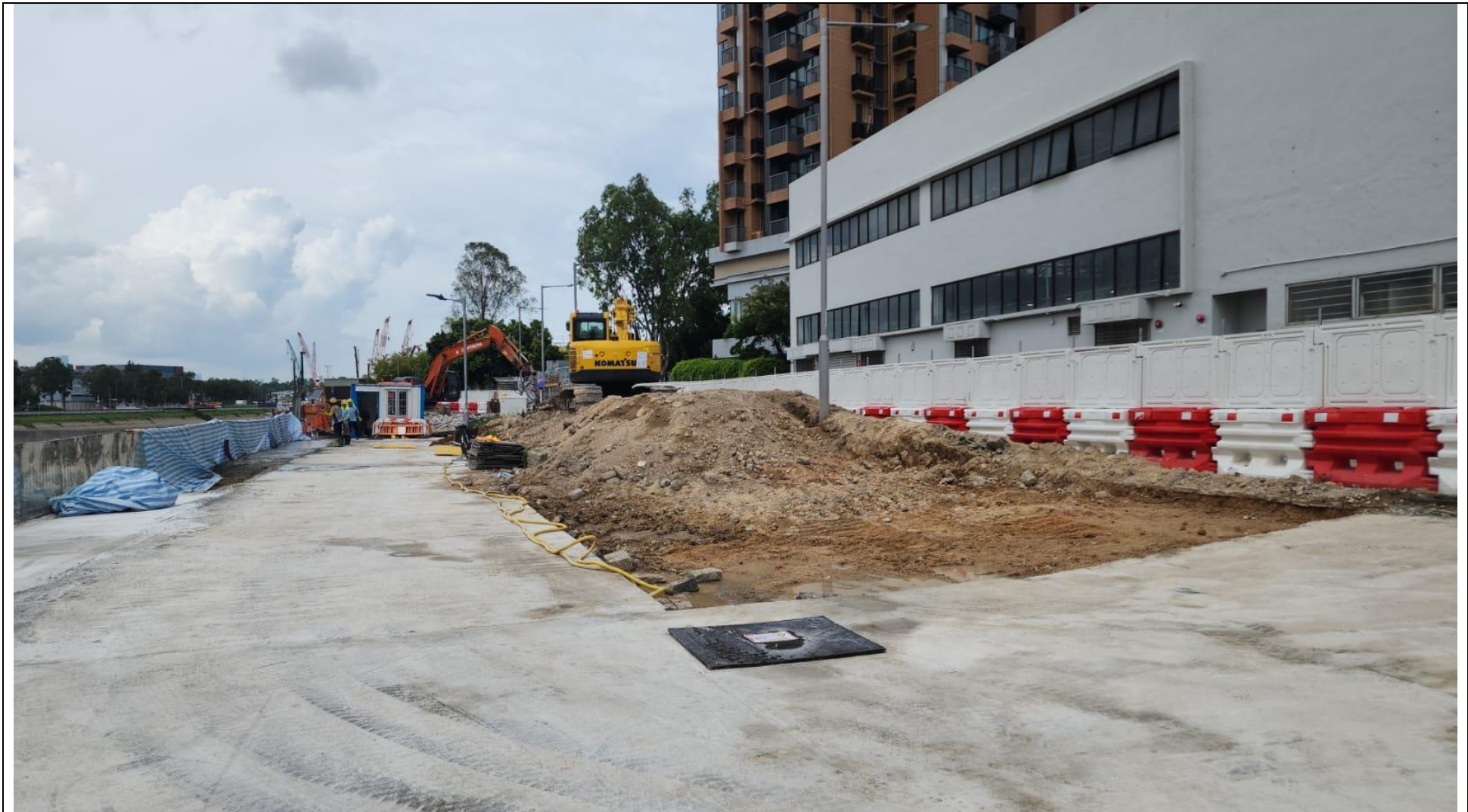
Photo 6 – Excavated materials outside the pumping station (Taken on 18 June 2024)
