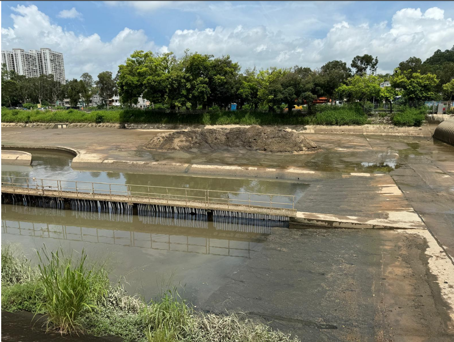
Photo 1 – Excavated sediment by DSD maintenance near OP3 (Taken on 18 June 2024)
