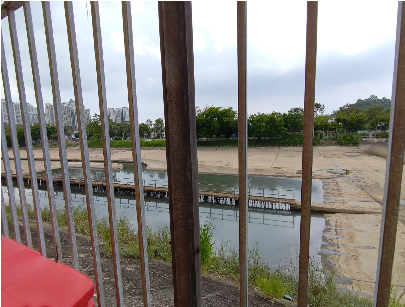
Photo 1 – Water retention pond managed by DSD (Photo taken on 12 September 2024)
