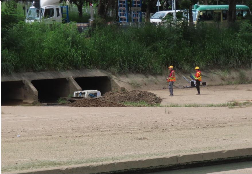
Photo 5: Dredging at section 3 of the Yuen Long Town Nullah
