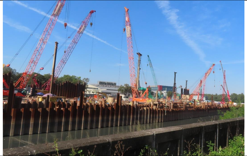
Photo 6: Sheet piling cofferdam construction at section 4 of the Yuen Long Town Nullah
