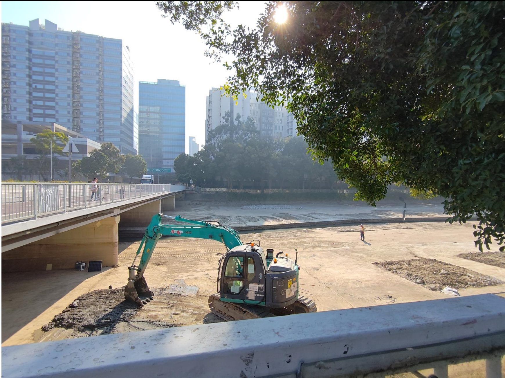
Photo 1 – Nullah works and sediment in the nullah
