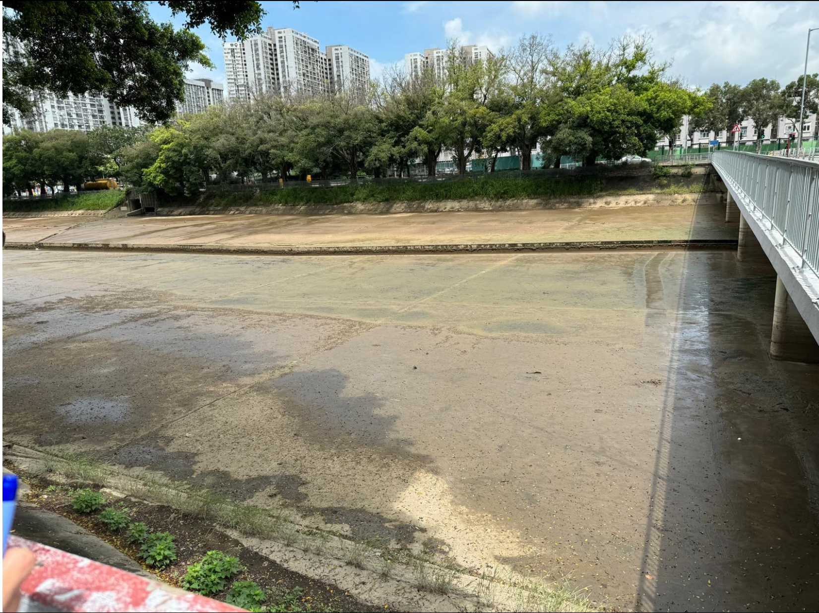
Photo 2 – Mud and sediment in the nullah near OP2 and OP4 (Taken on 18 June 2024)
