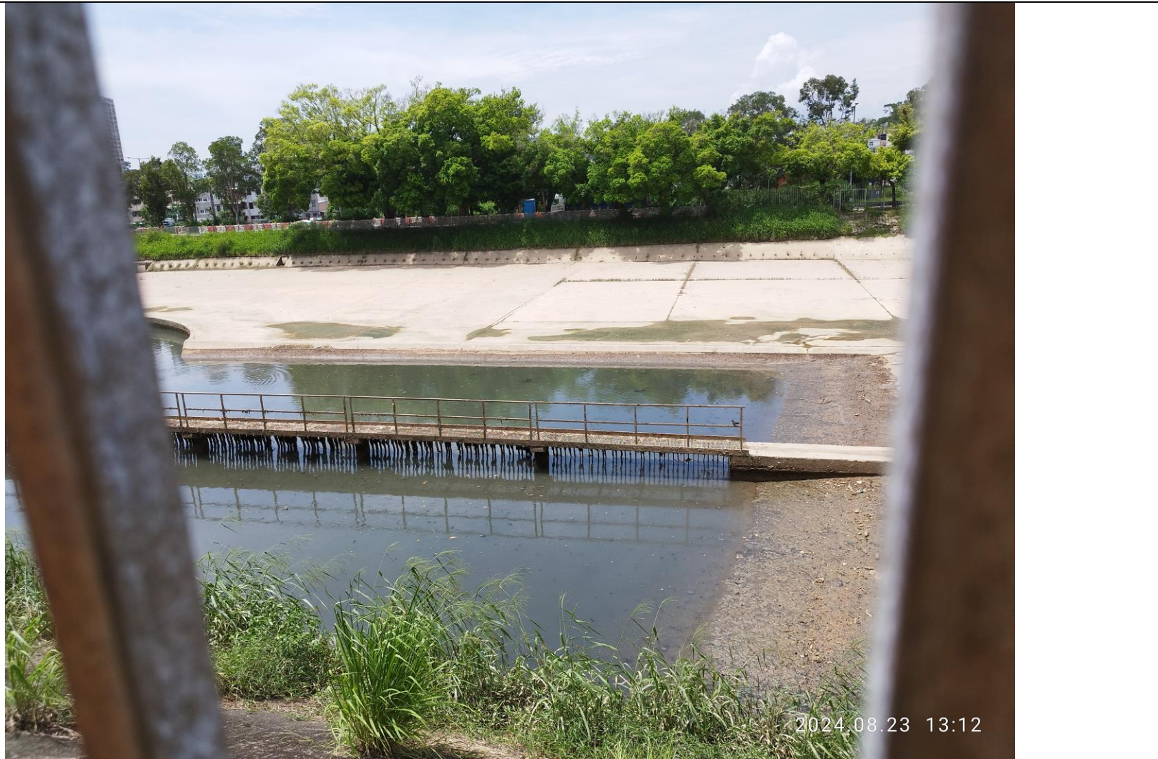
Photo 1 – Water retention pond managed by DSD (Photo taken on 23 August 2024)
