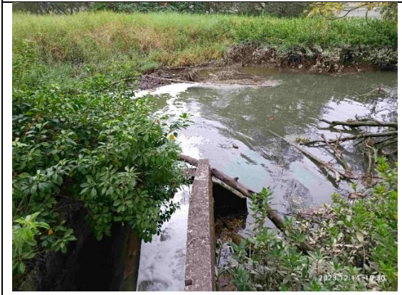
Photo 13. Water gate outflow point
