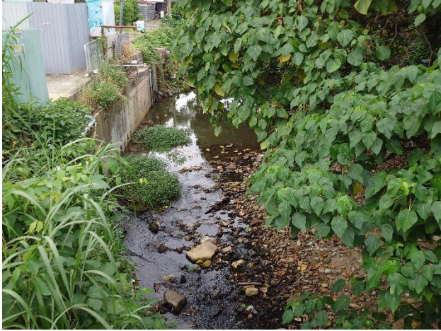
Potential receptor site A at Lin Fa Tei Date taken: 9 th November 2023
