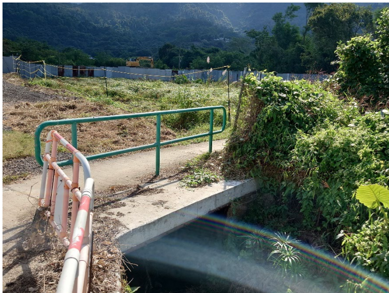
Plate 5. Covered portion of CH.B0.00 – CH.B149.77 on 22 November 2023.
