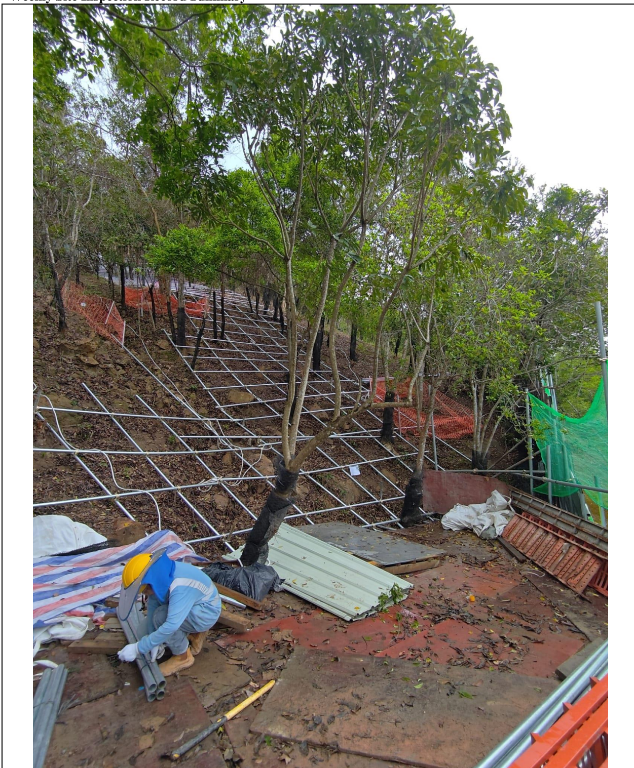
Photo 2: Site photo of Catchment B
