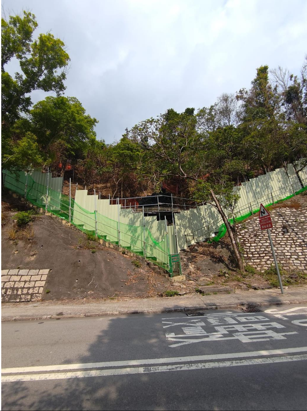
Photo 2: Site photo of Catchment B
