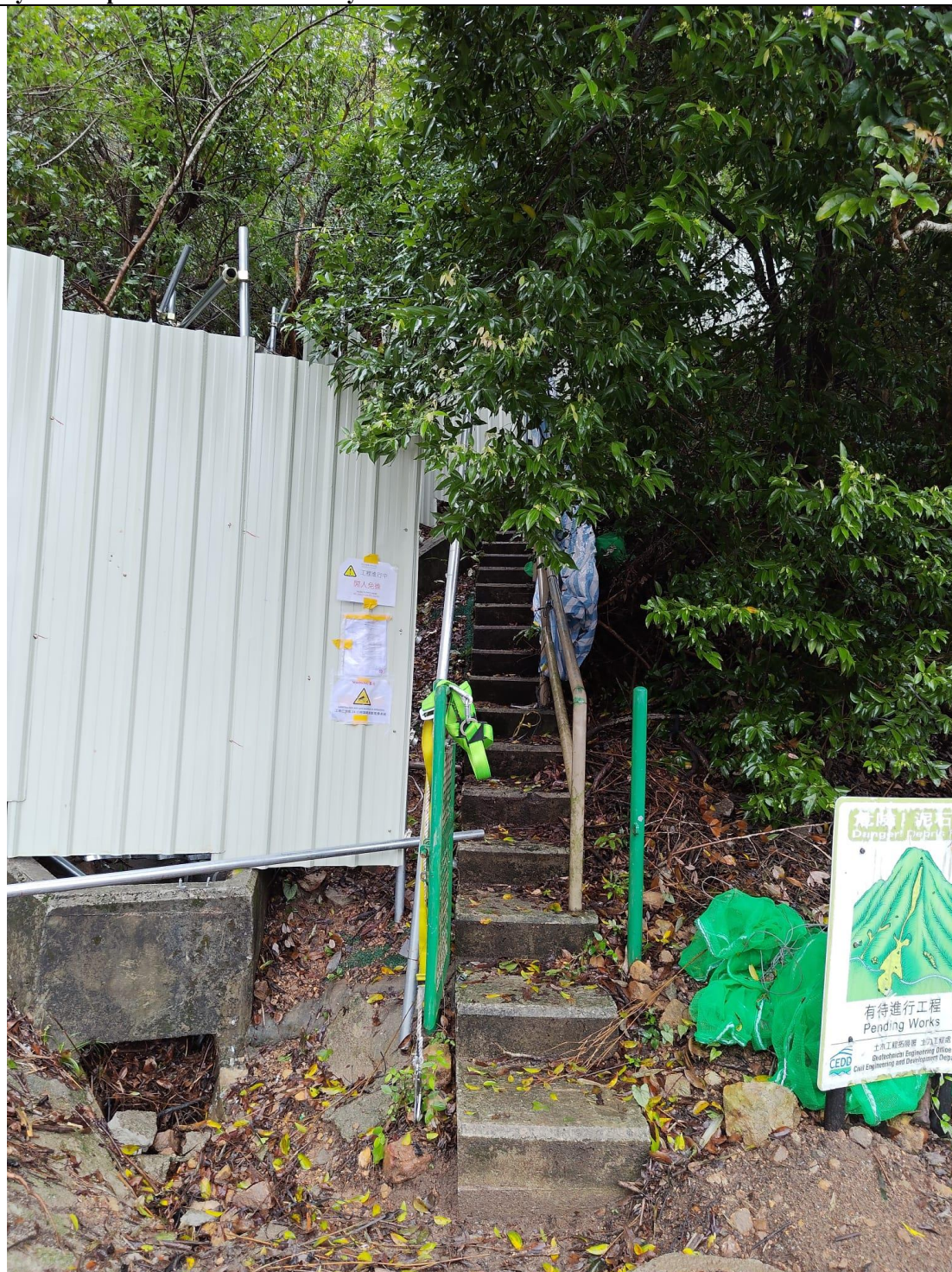
Photo 2: Site photo of Catchment C
