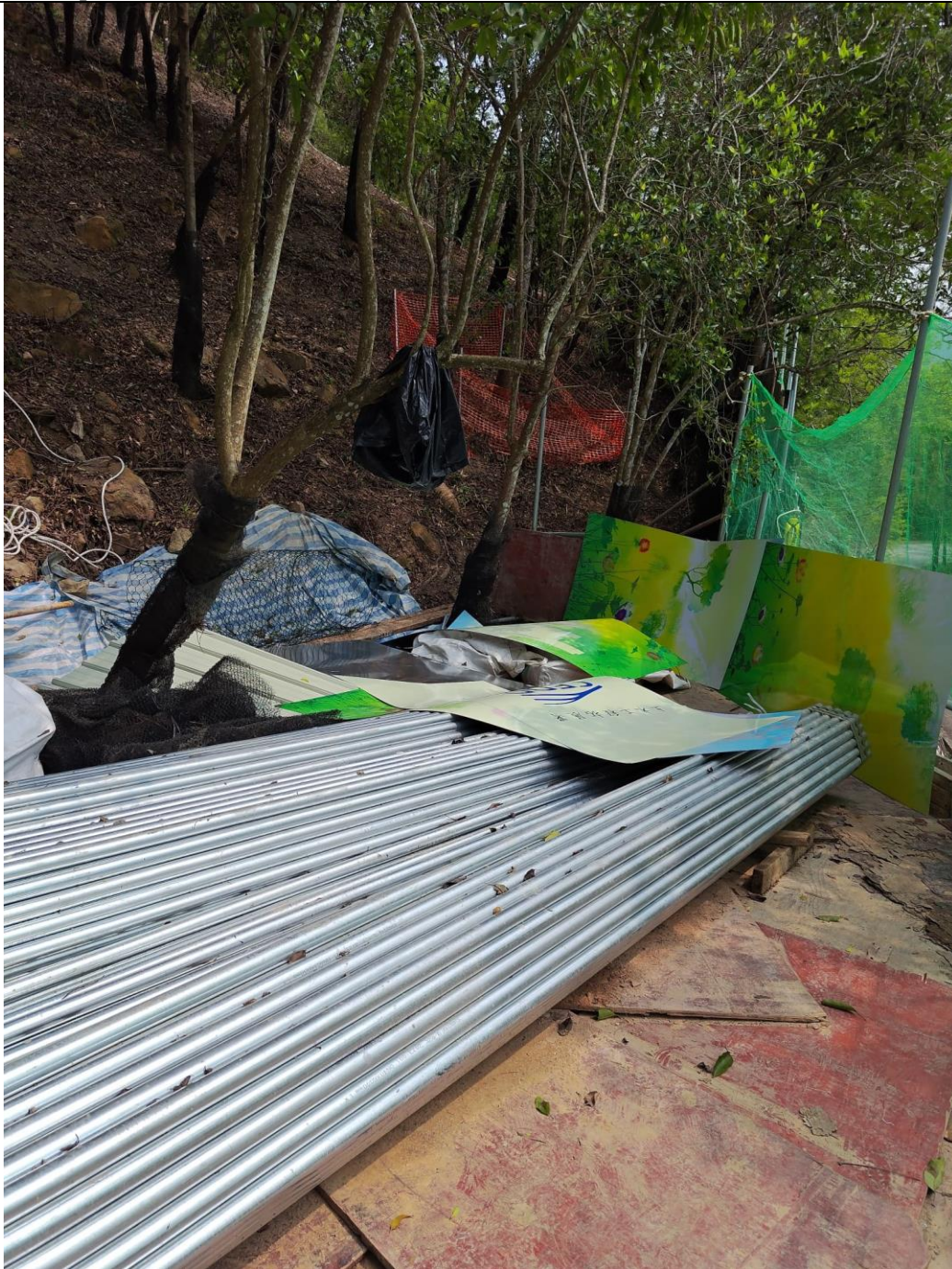
Photo 2: Site photo of Catchment B
