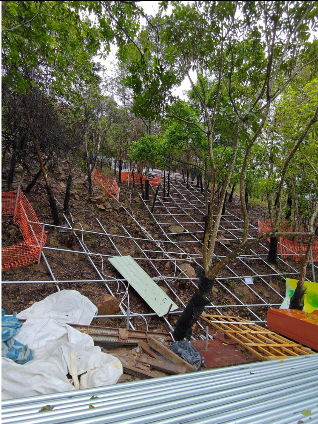
Photo 2: Site photo of Catchment B
