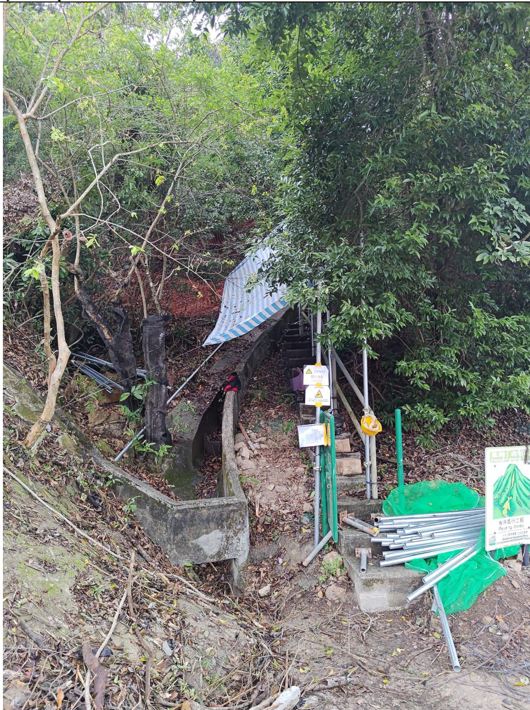
Photo 2: Site photo of Catchment C
