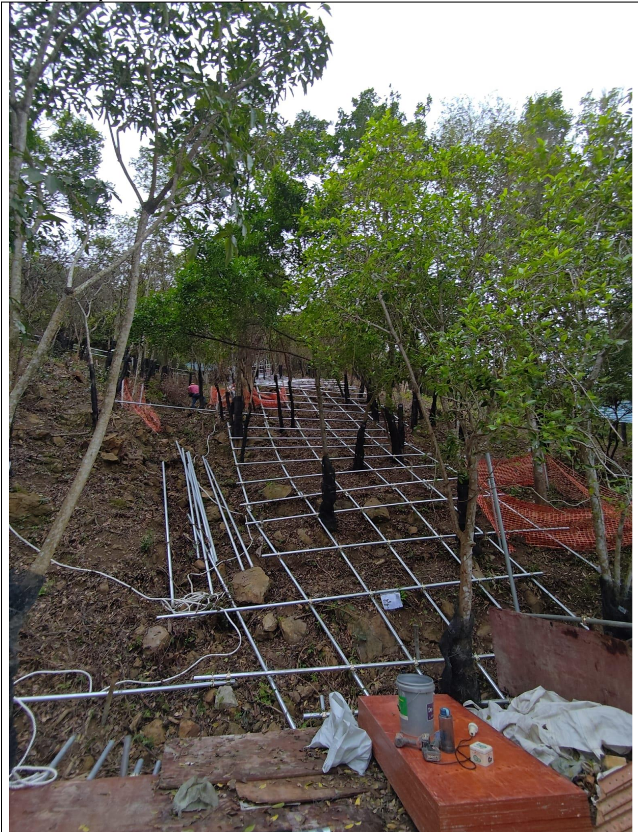
Photo 2: Site photo of Catchment B
