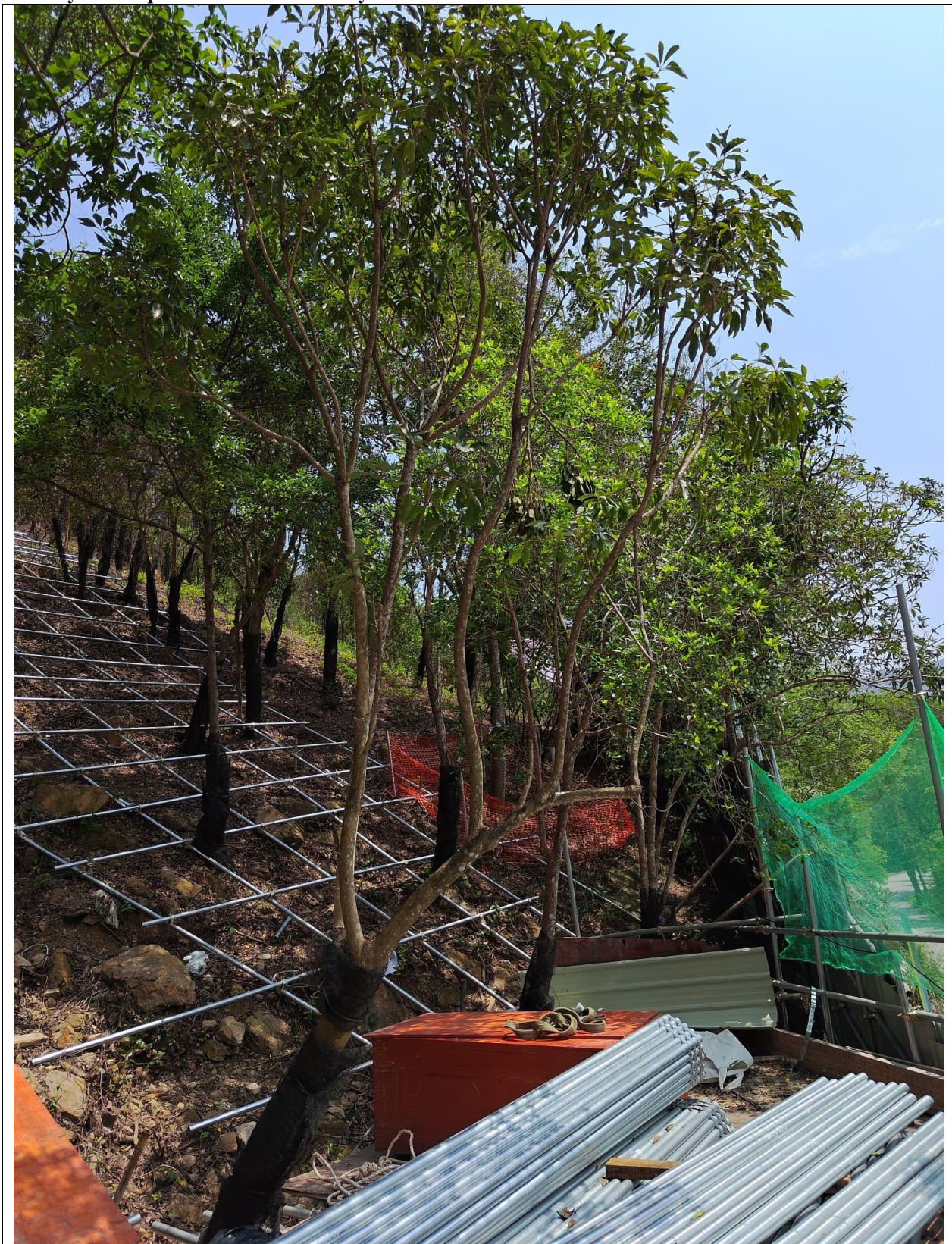
Photo 2: Site photo of Catchment B
