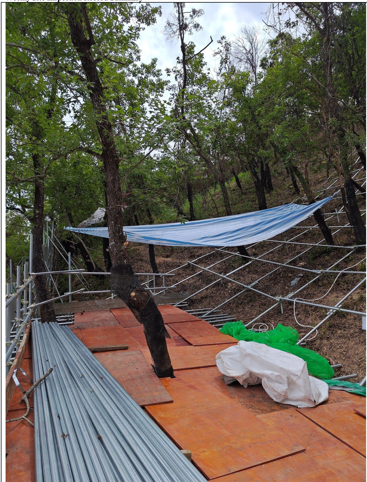
Photo 2: Site photo of Catchment C
