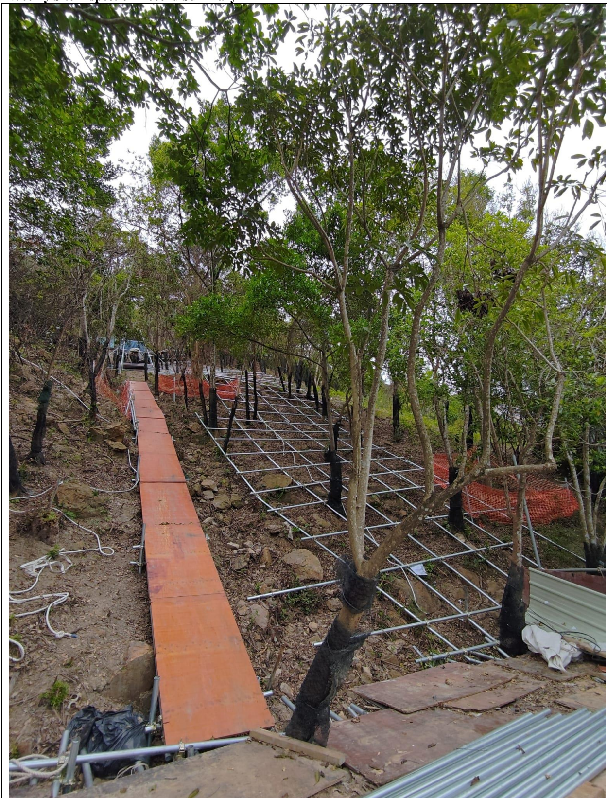
Photo 2: Site photo of Catchment B
