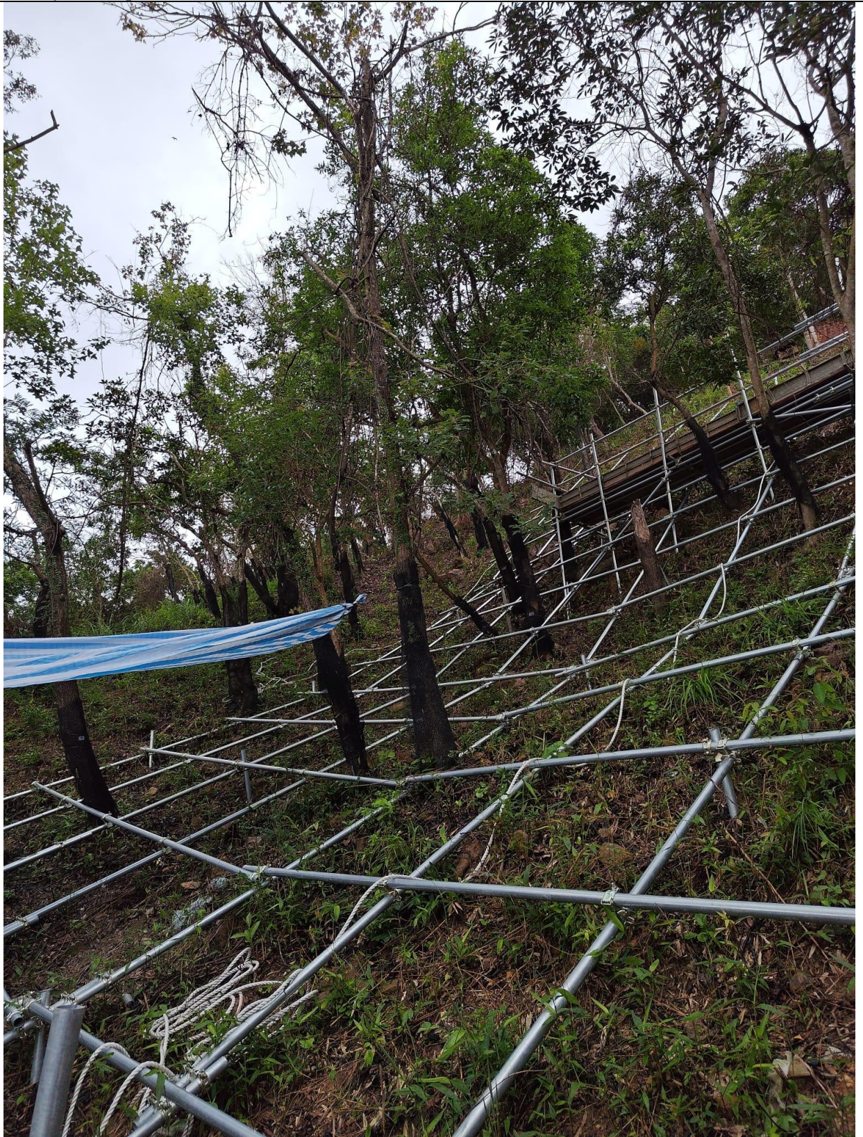
Photo 2: Site photo of Catchment C
