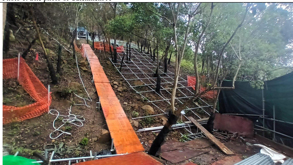
Photo 2: Site photo of Catchment B
