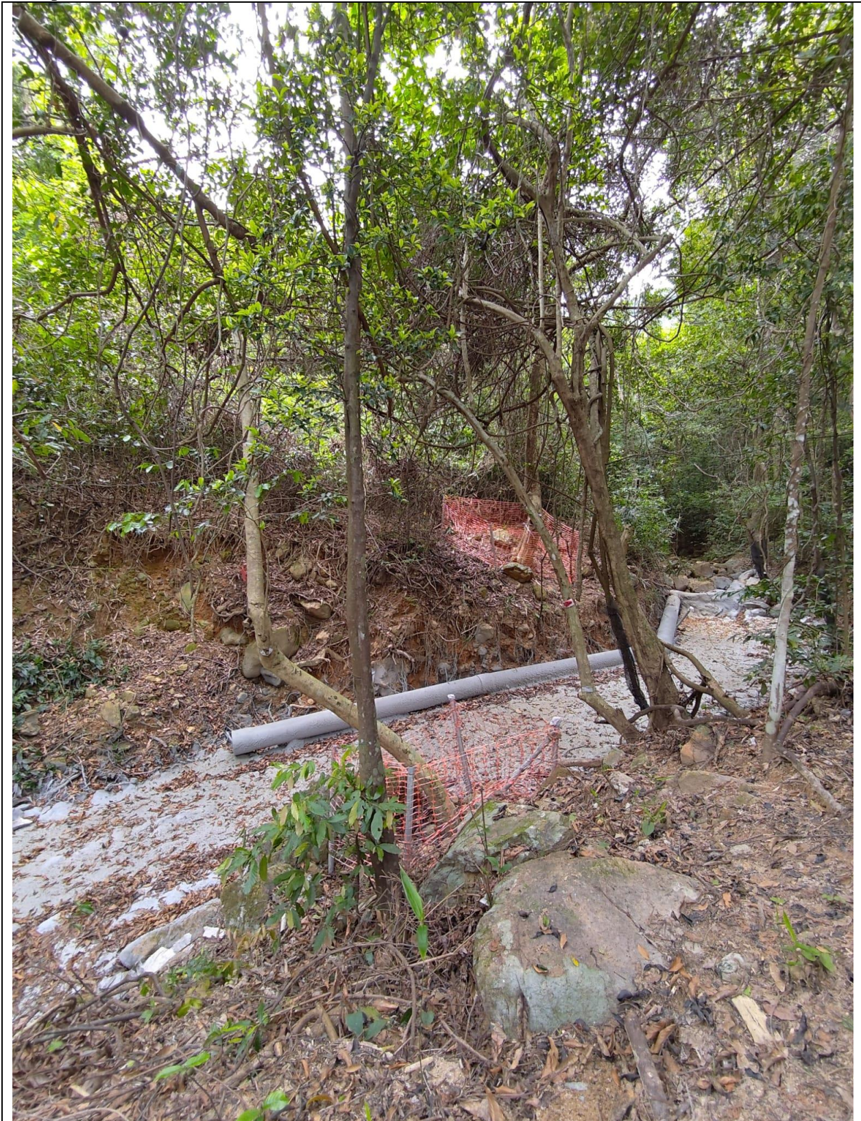
Photo 1: Site photo of Catchment A
