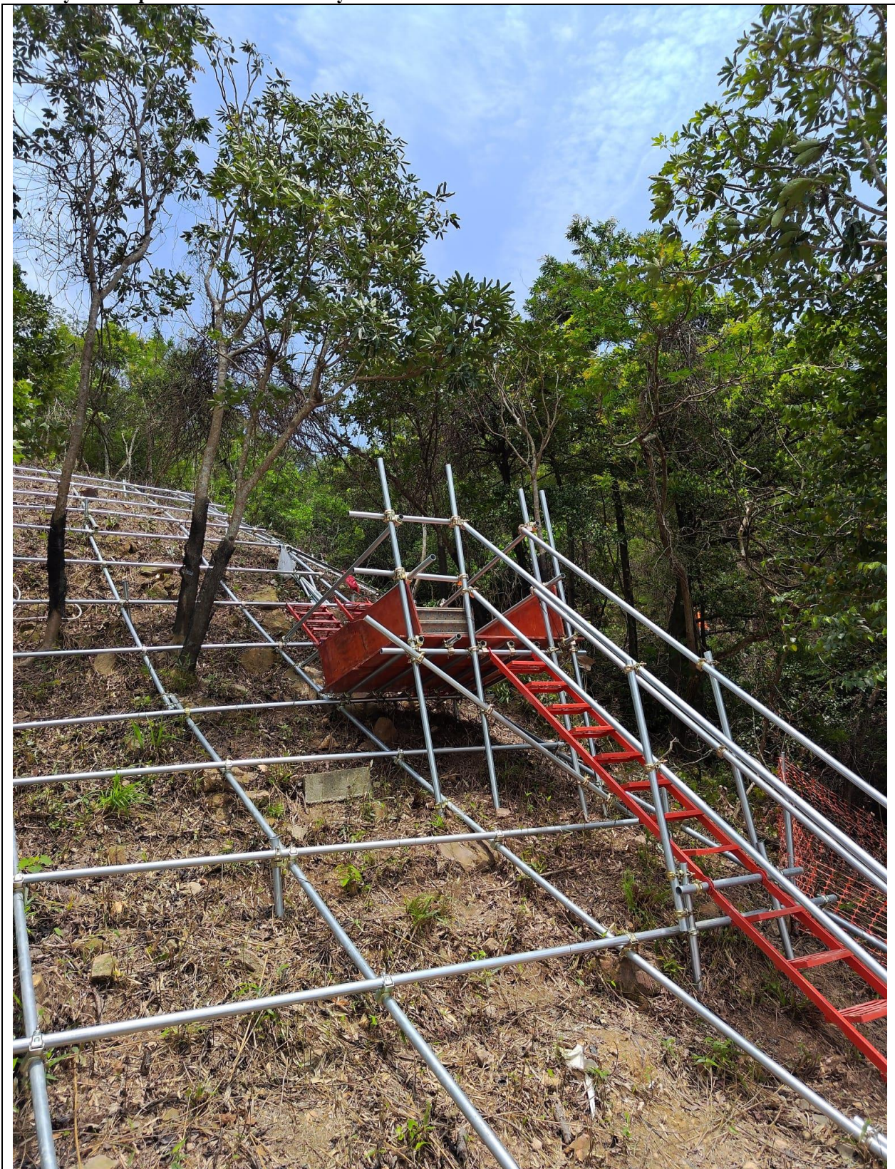
Photo 2: Site photo of Catchment C
