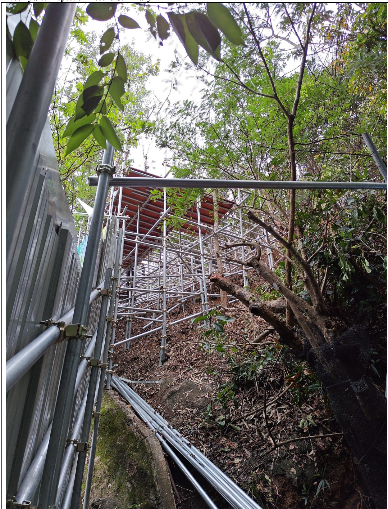
Photo 2: Site photo of Catchment C
