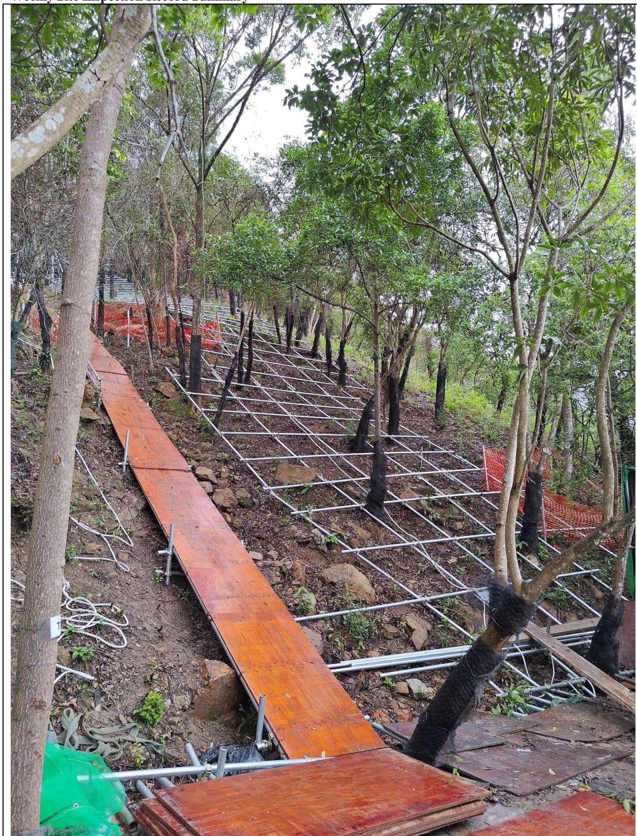
Photo 2: Site photo of Catchment B
