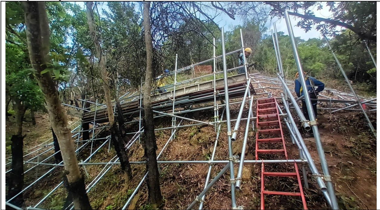
Photo 2: Site photo of Catchment C
