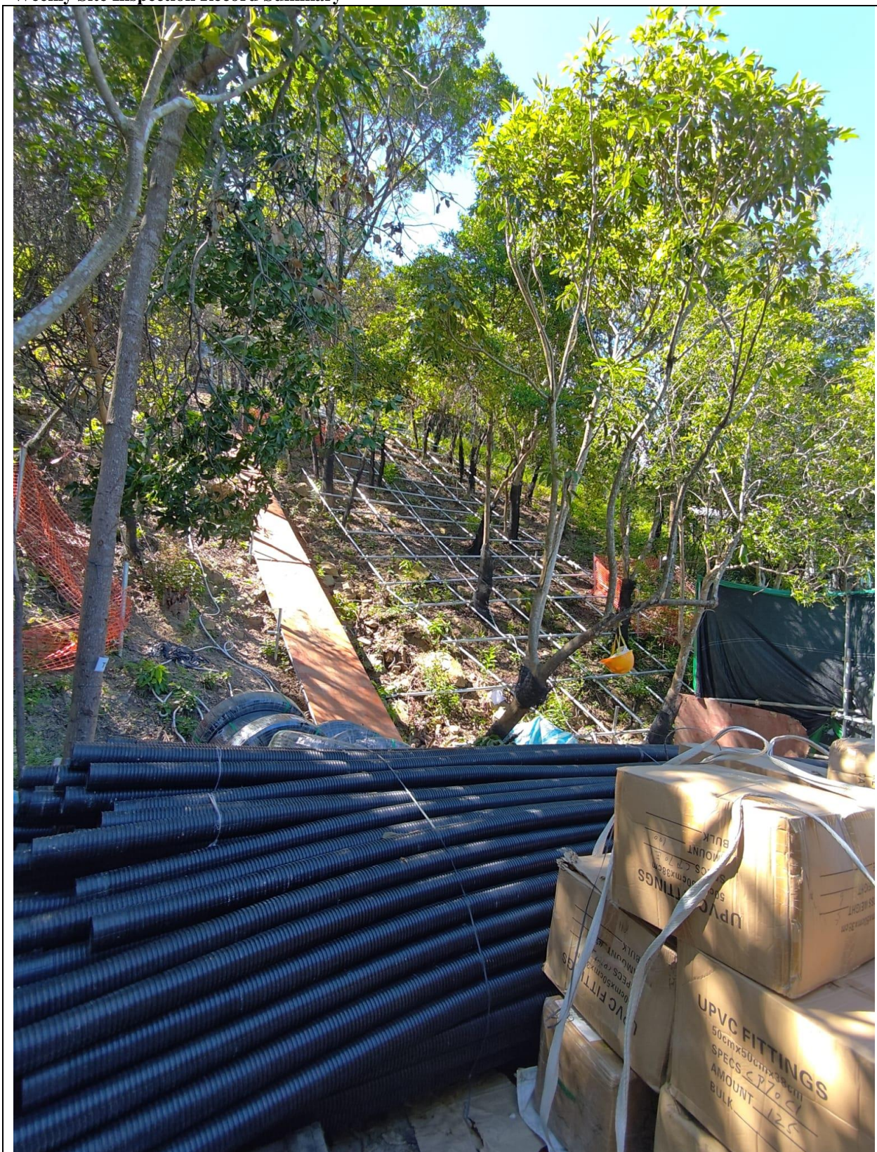
Photo 2: Site photo of Catchment B
