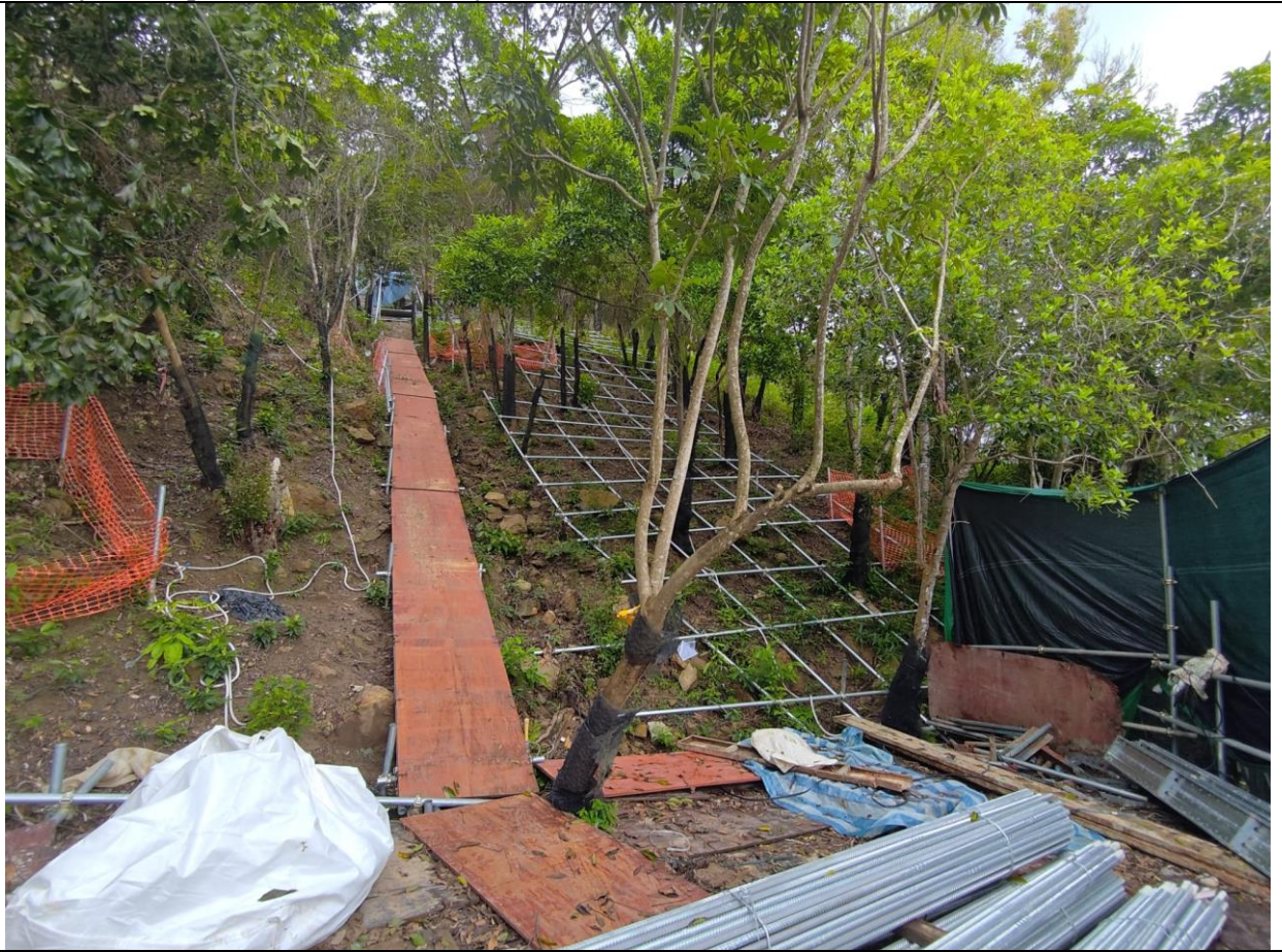
Photo 2: Site photo of Catchment B
