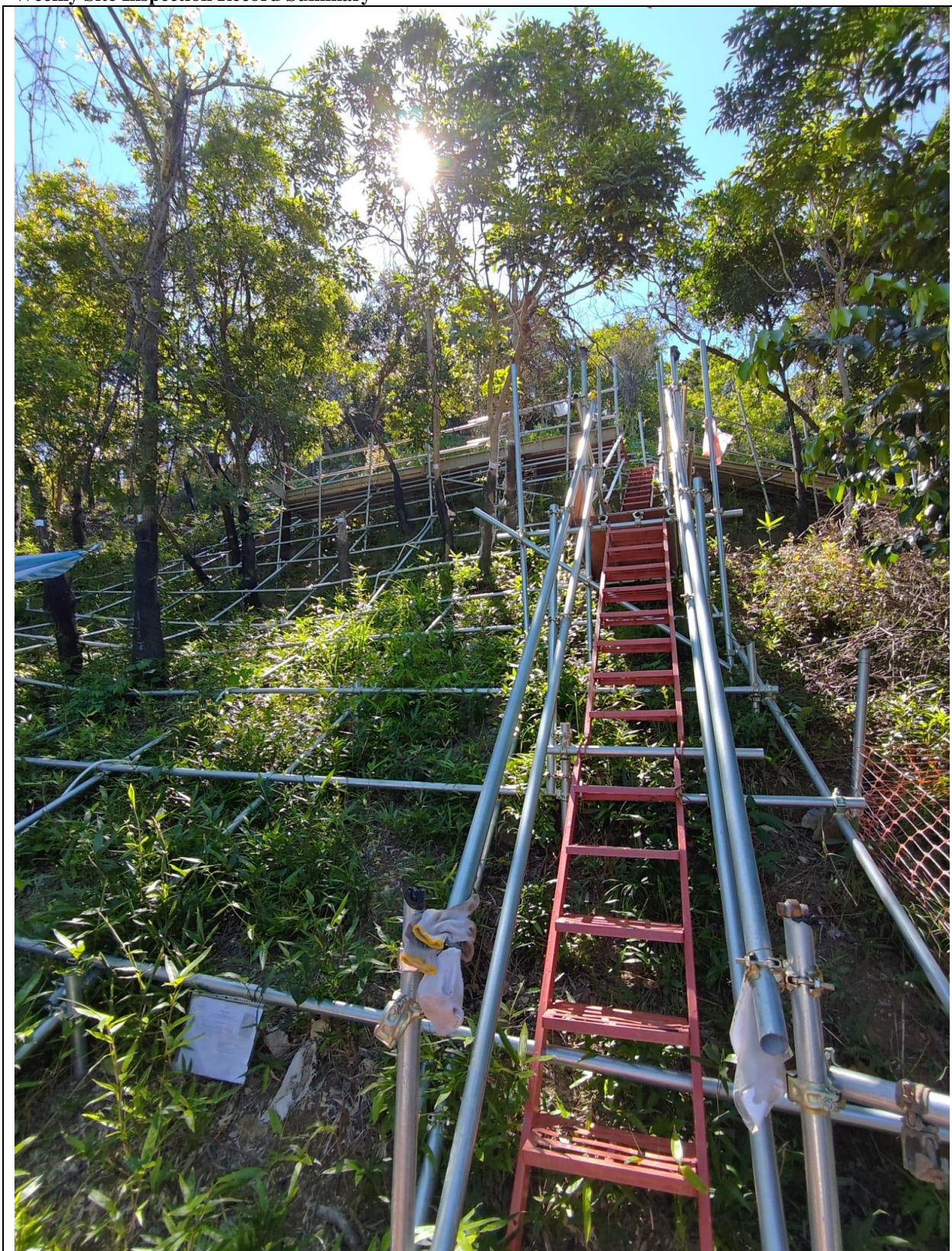
Photo 2: Site photo of Catchment C
