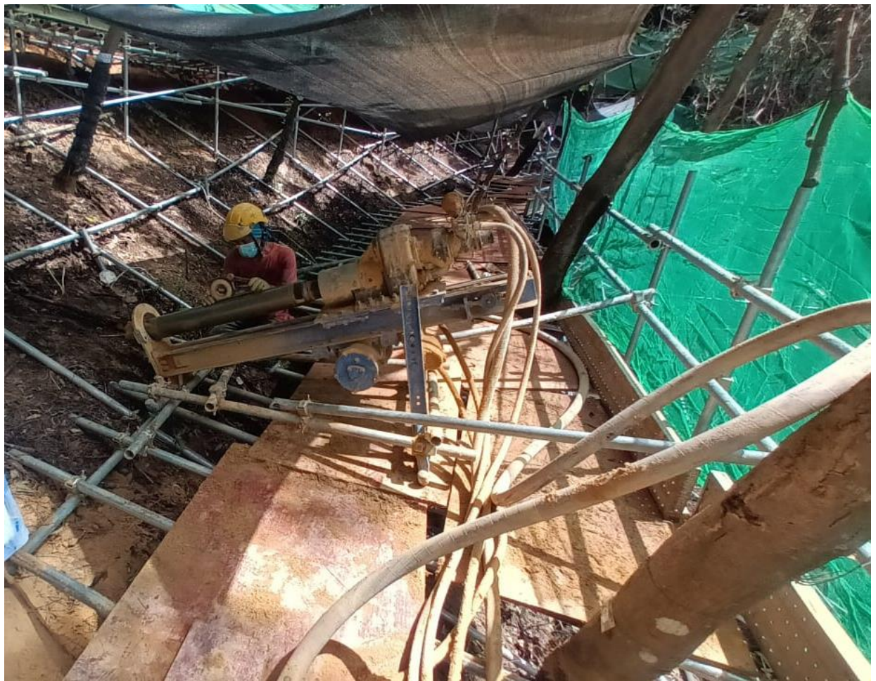
Photo 4: Site photo during soil nail process inside catchment B
