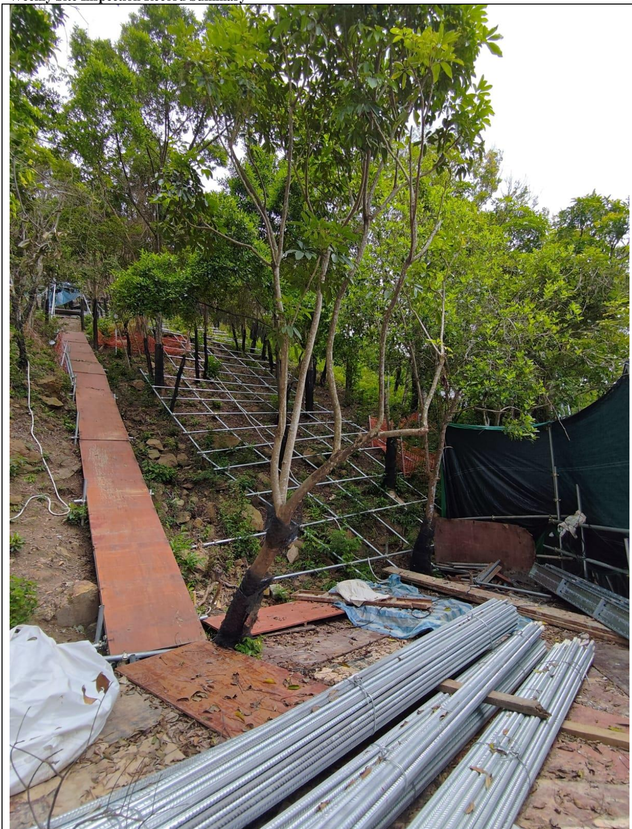
Photo 2: Site photo of Catchment B
