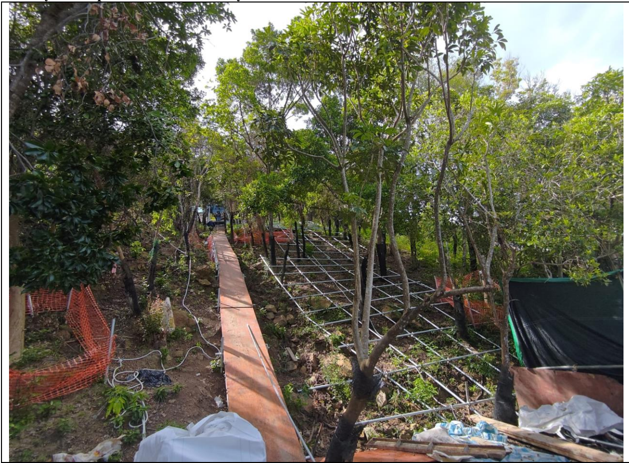
Photo 2: Site photo of Catchment B
