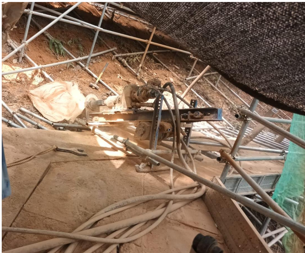
Photo 4: Site photo during soil nail process inside catchment B
