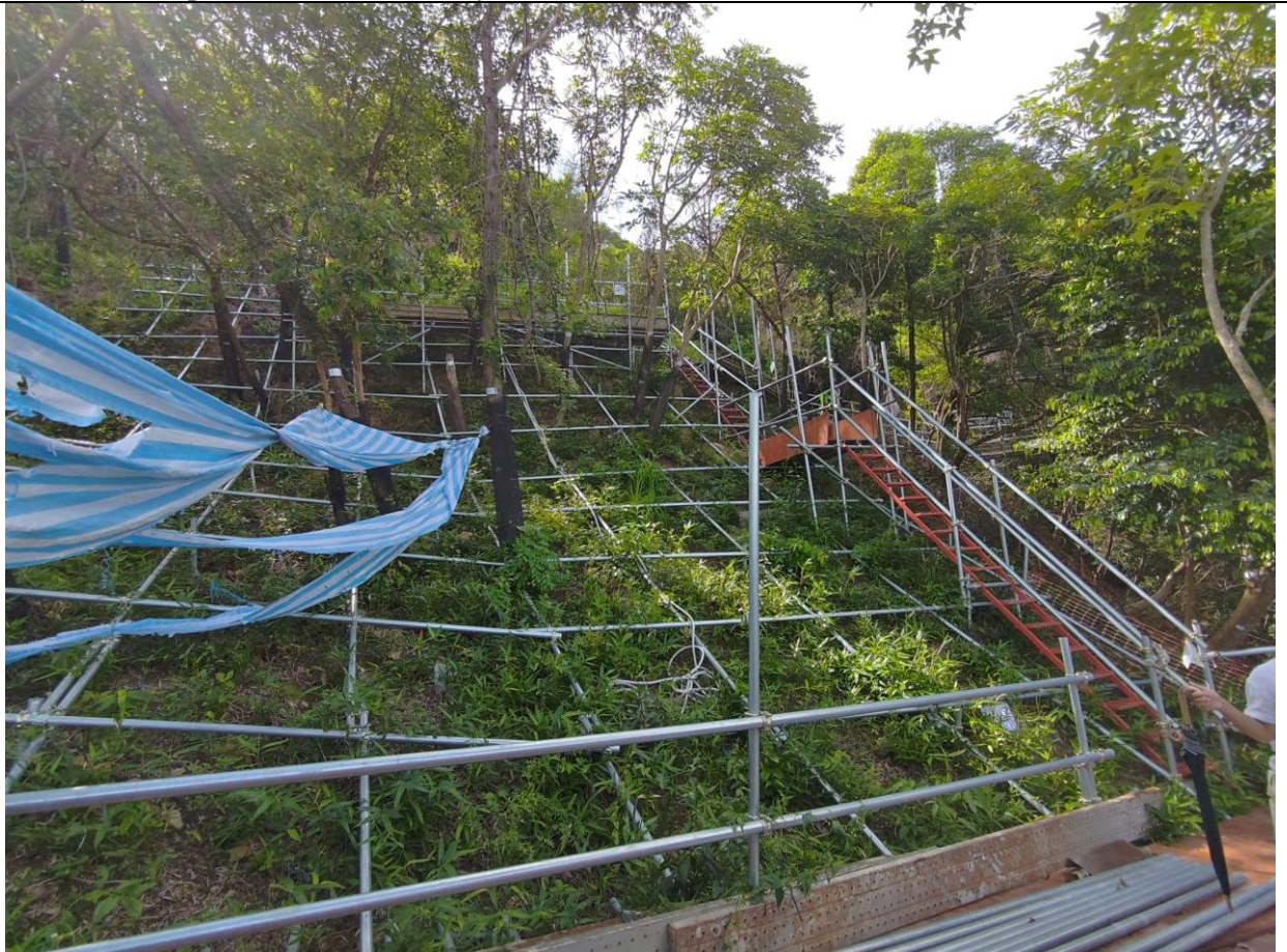
Photo 2: Site photo of Catchment C
