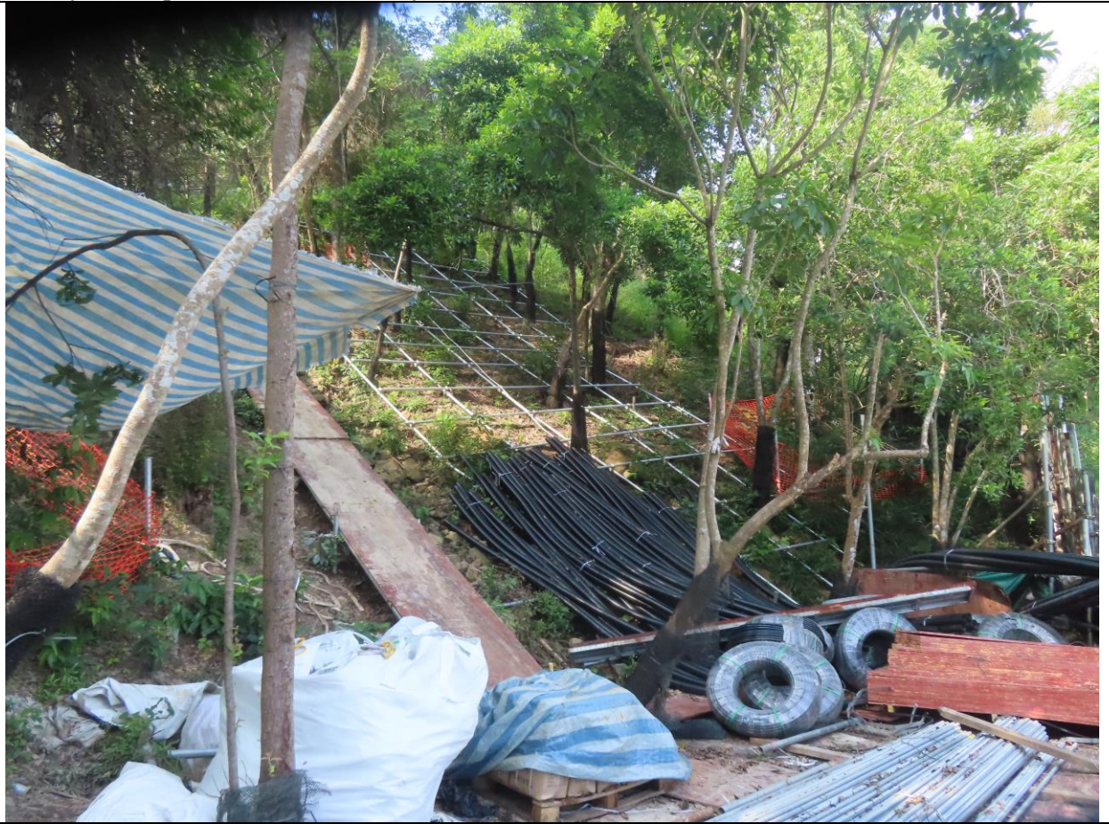
Photo 2: Site photo of Catchment B
