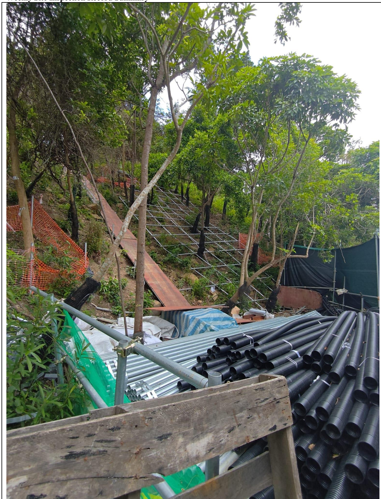
Photo 2: Site photo of Catchment B
