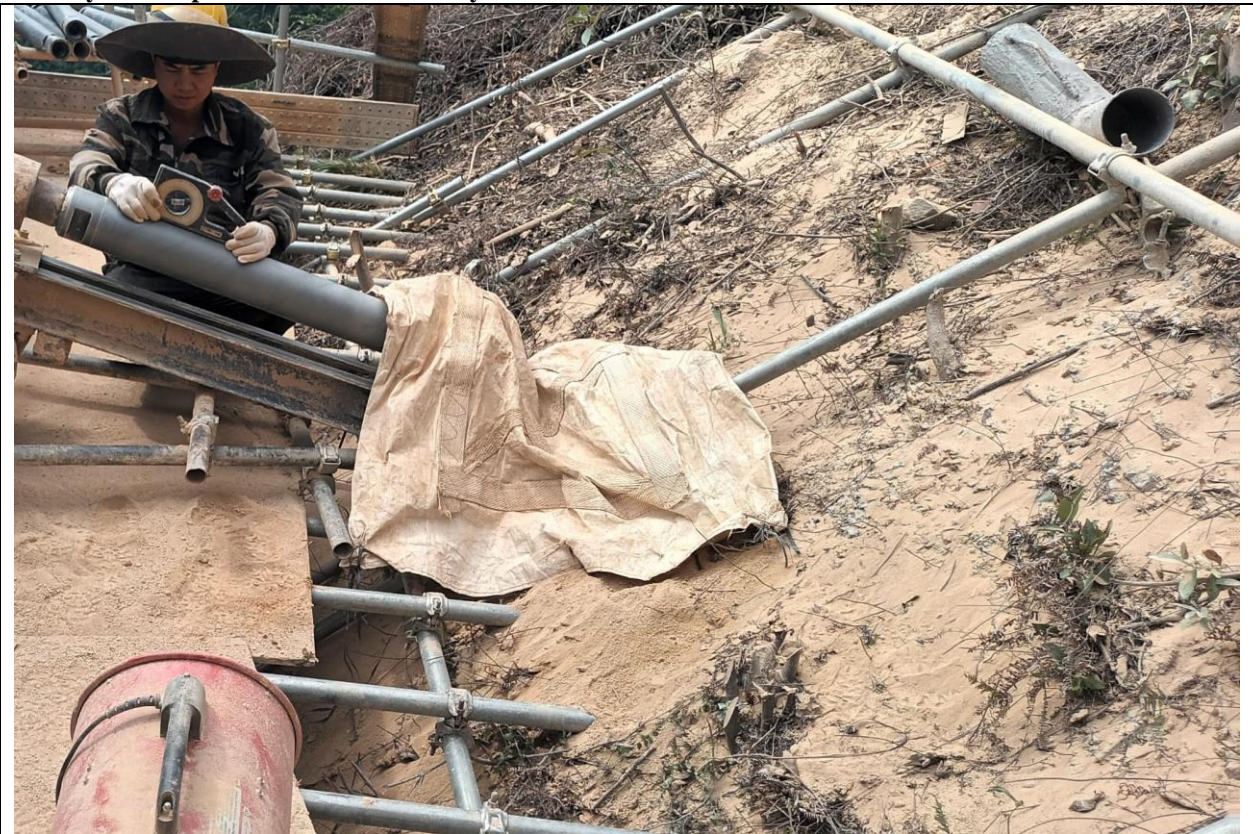
Photo 4: Site photo during soil nail process
