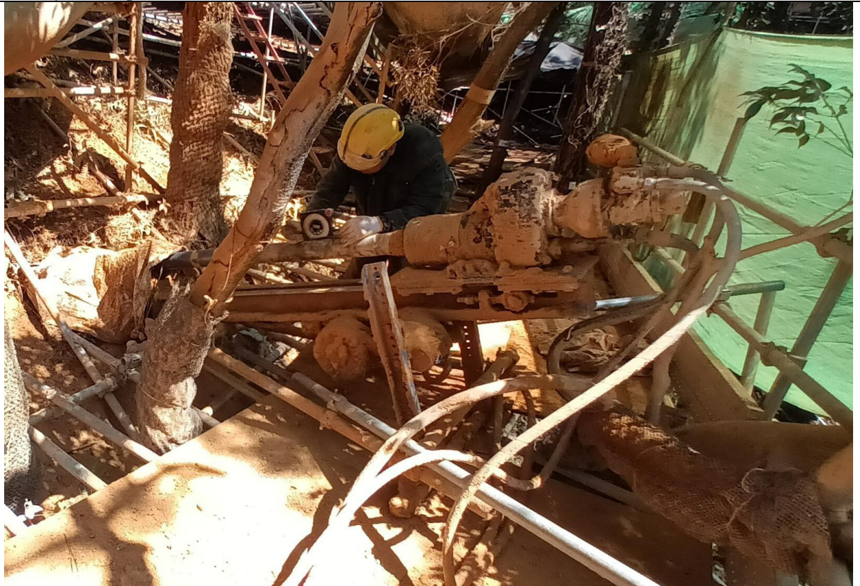
Photo 4: Site photo during soil nail process
