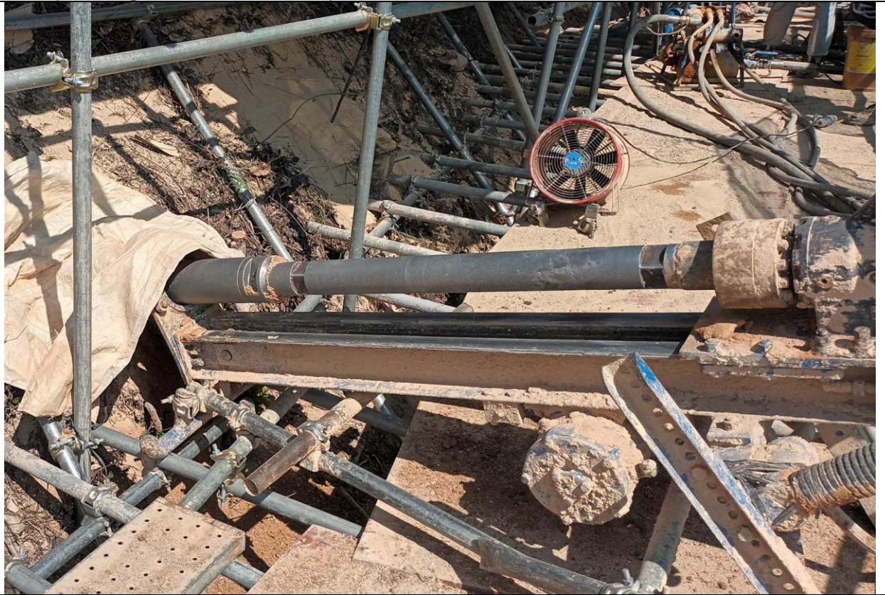
Photo 4: Site photo during soil nail process
