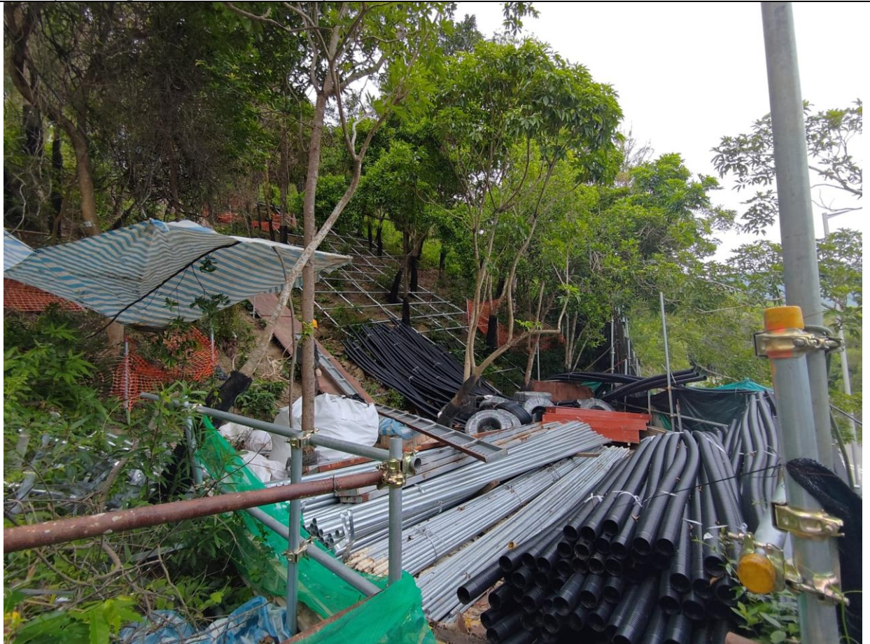
Photo 2: Site photo of Catchment B
