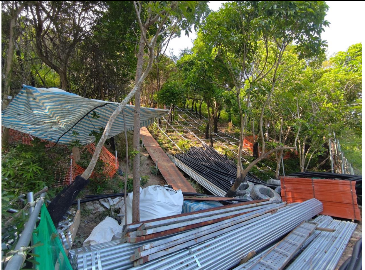
Photo 2: Site photo of Catchment B
