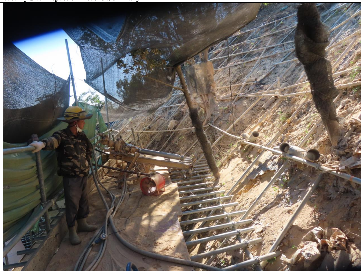
Photo 4: Site photo during soil nail process
