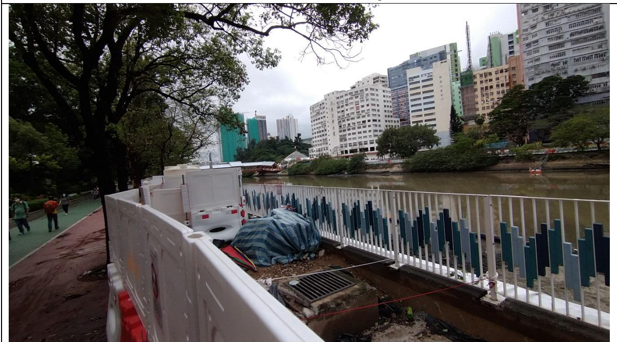
Site preparation works along Tuen Mun River Channel
