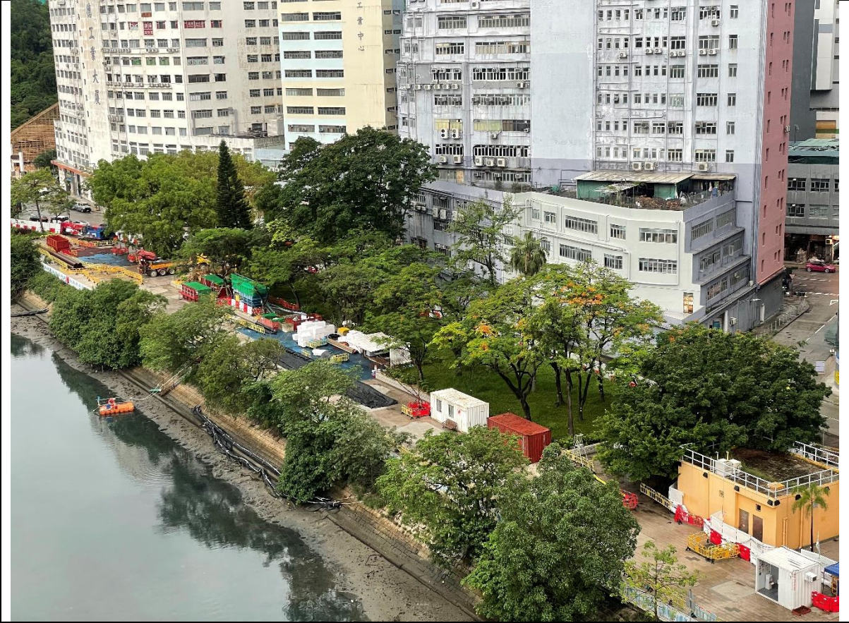
Site preparation works along Tuen Mun River Channel
