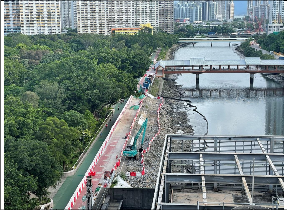
Site preparation works along Tuen Mun River Channel and construction of temporary platform
