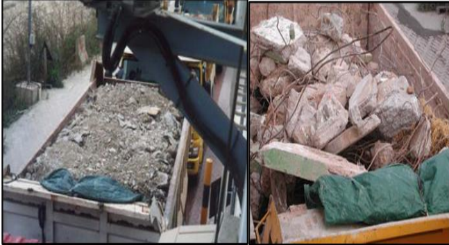
Sorted broken concrete materials to be delivered to recycling facilities
