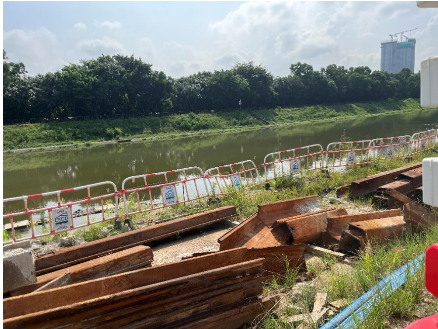
Sheet-piling (Non-project-related, taken on 02 September 2024)
