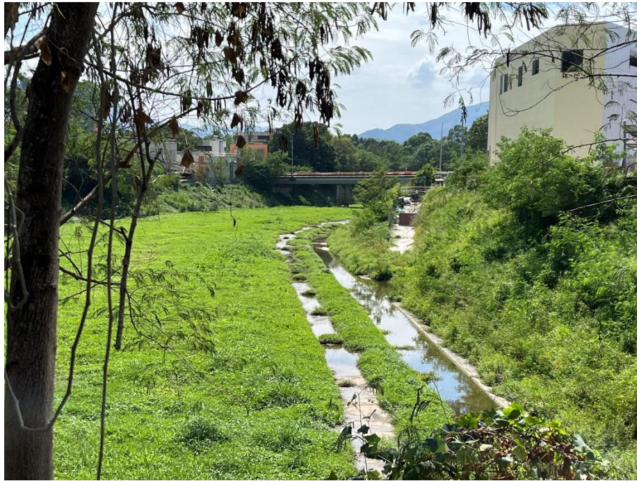
Shek Sheung River (Taken on 16 October 2024)
