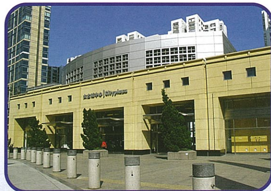
Acoustic enclosures for chillers, City Plaza, Hong Kong
