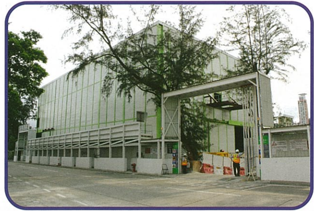
Wylie Road Ancillary Building, Hong Kong
