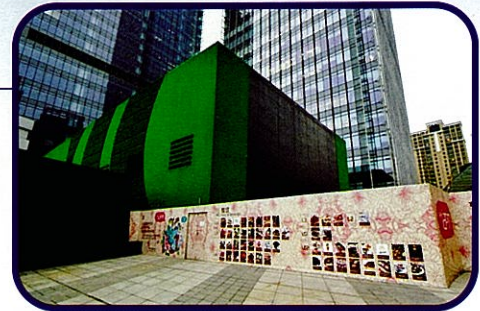
Shanghai IAPM Mall, Huaihai Road Central, China
