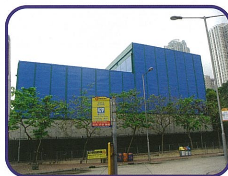
MTR Access Shafts at KET Praya
