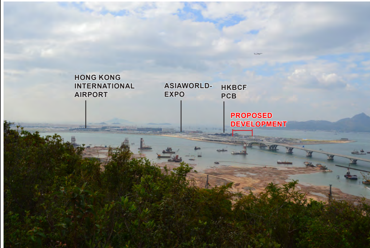
Existing Baseline Condition
