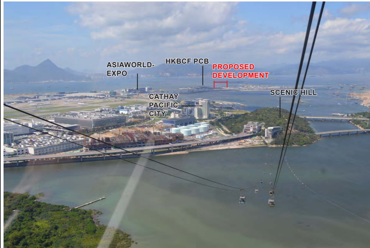
Existing Baseline Condition
