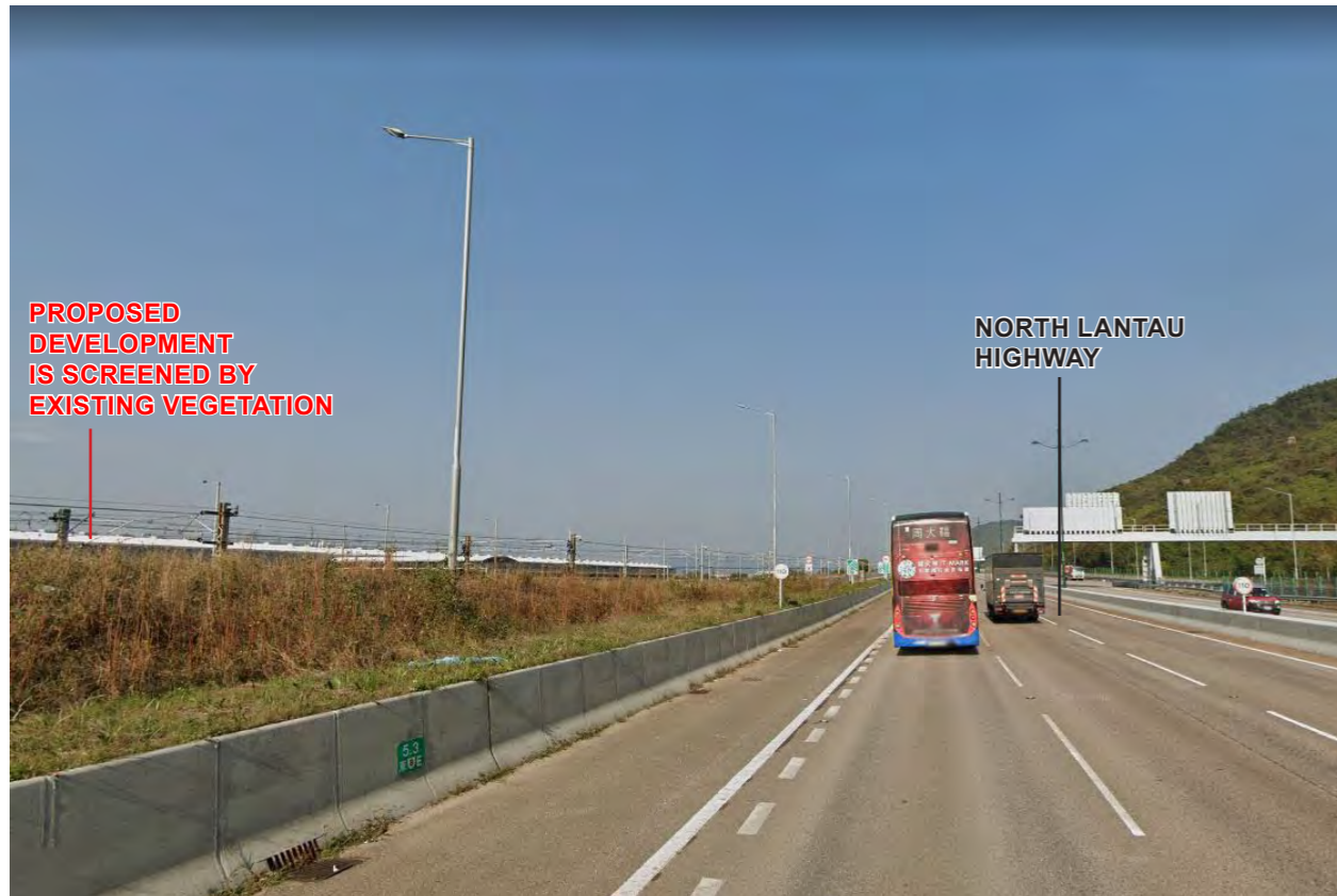
Existing Baseline Condition
