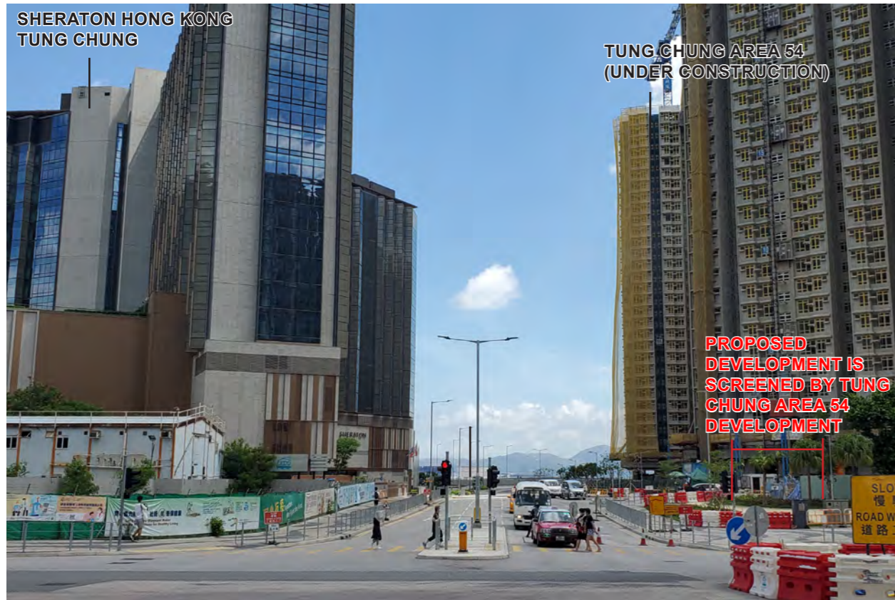
Existing Baseline Condition
