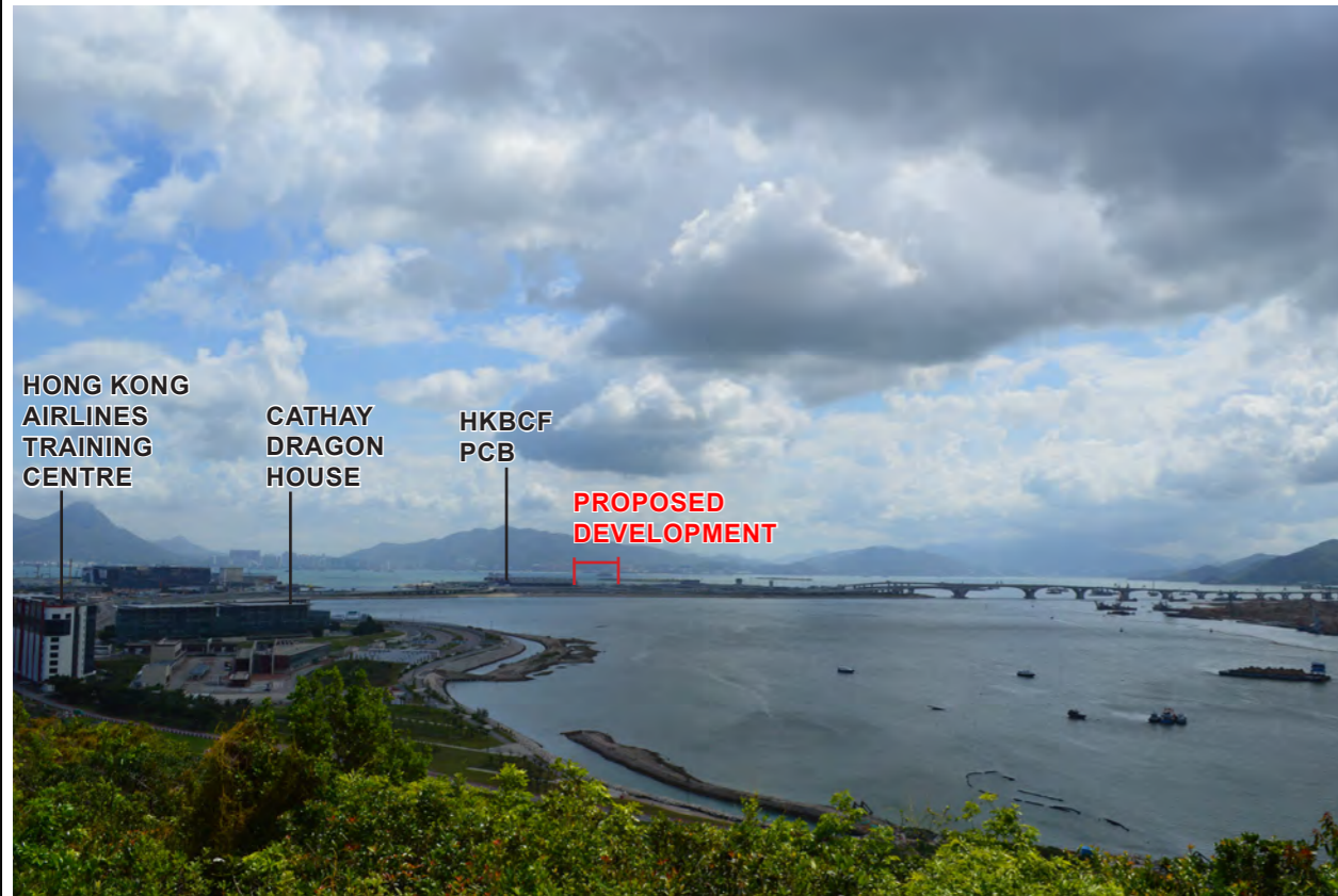
Existing Baseline Condition
