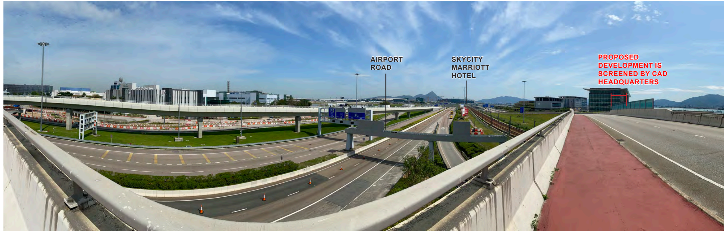
Proposed Development with Mitigation Measures (Day 1 of Operational Stage)
