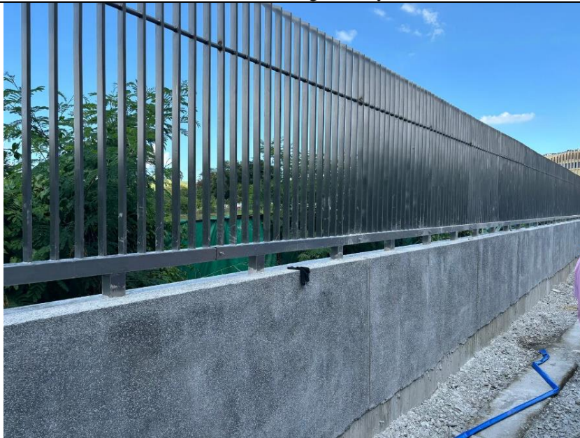
Construction of fence wall
