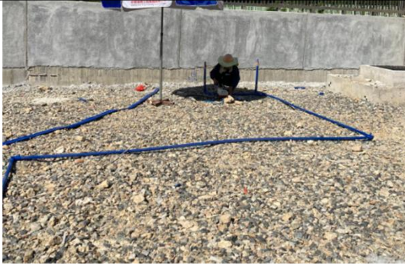
Installation of Irrigation System
