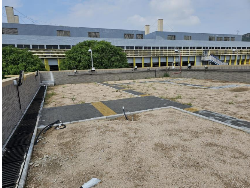
Soil filling for planting works at HCF Roof
