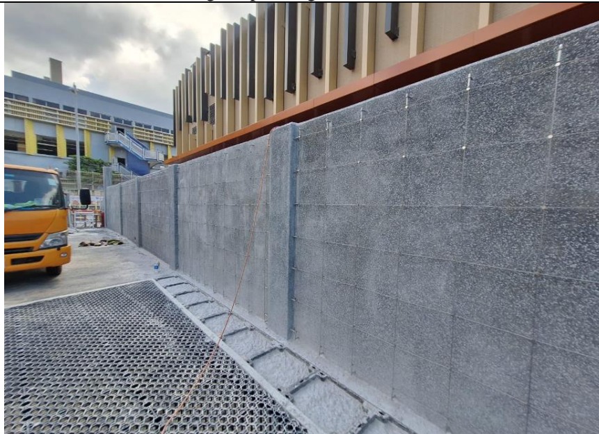
Installation of Vertical Green Mesh
