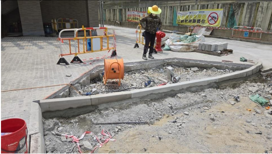
Installation of Drop Kerb
