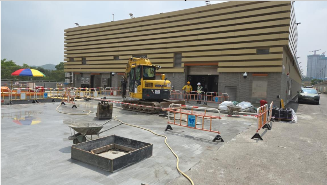
Removal of EVA Temporary Bitumen
