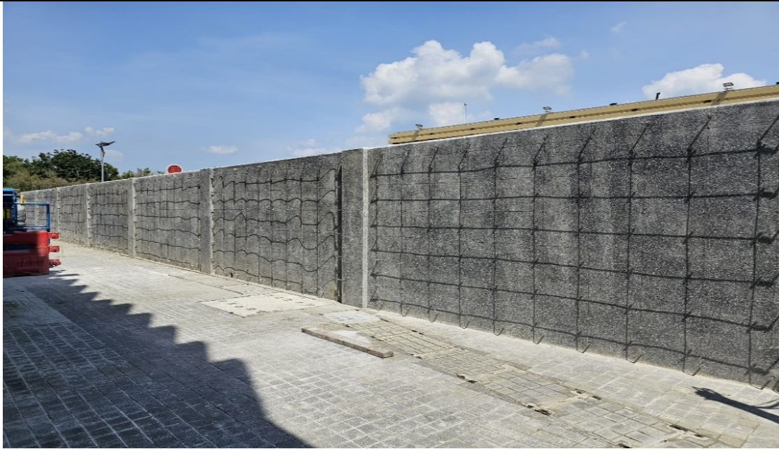
Installation of Vertical Green Mesh
